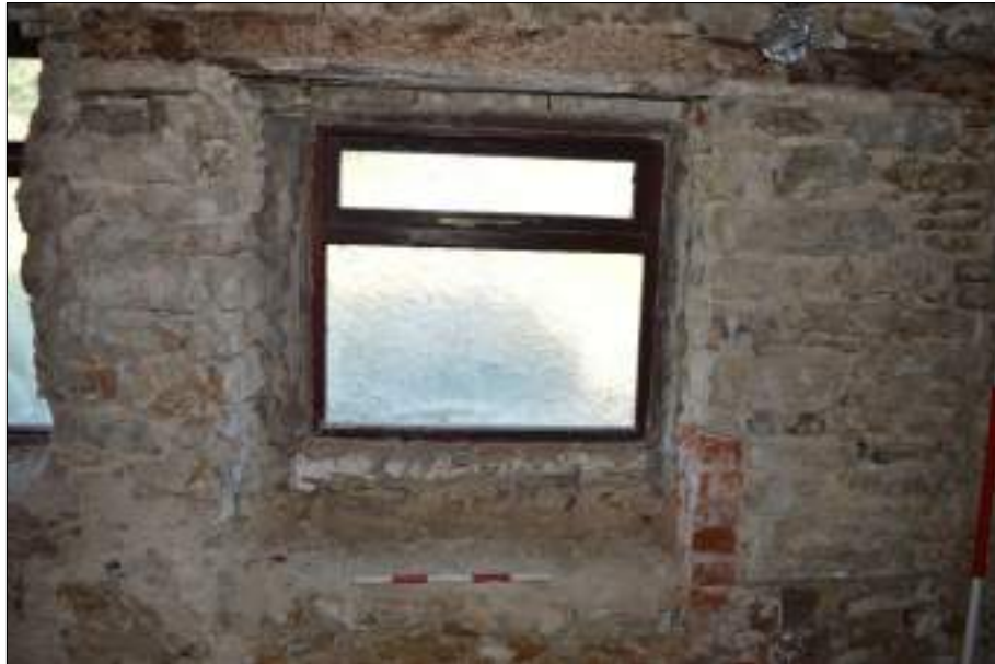
Plate 45 (shot 71): Detail of window, northwestern wall, Room 3, 0.5m scale
