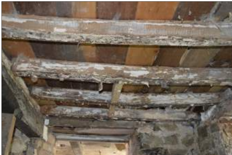
Plate 42 (shot 75): Detail of ceiling, Room 3, no scale
