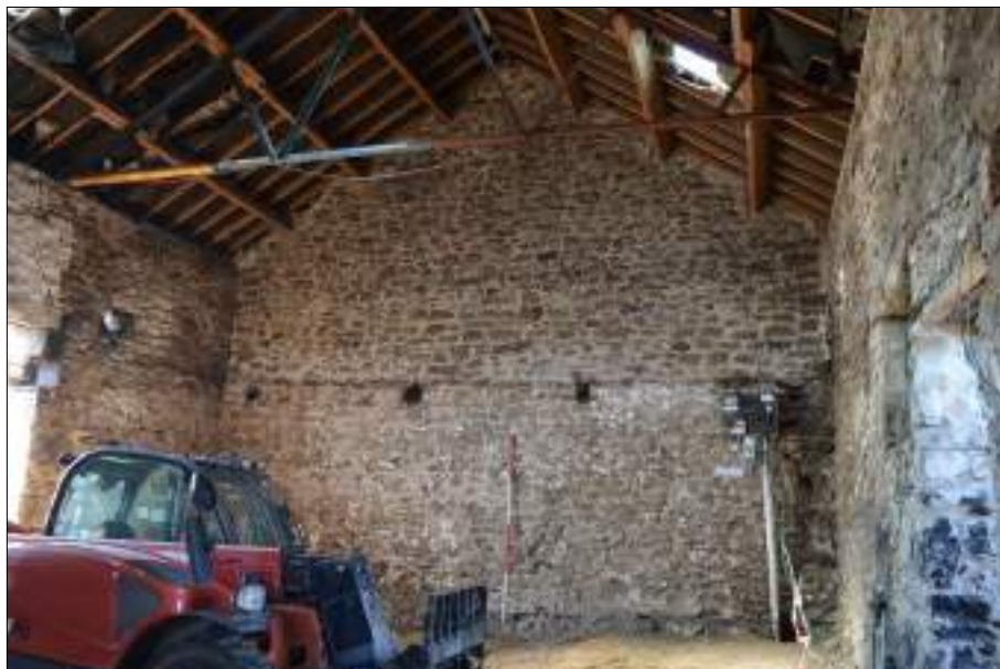
Plate 91 (shot 106): Southwestern wall of Room 6, 2m scale
