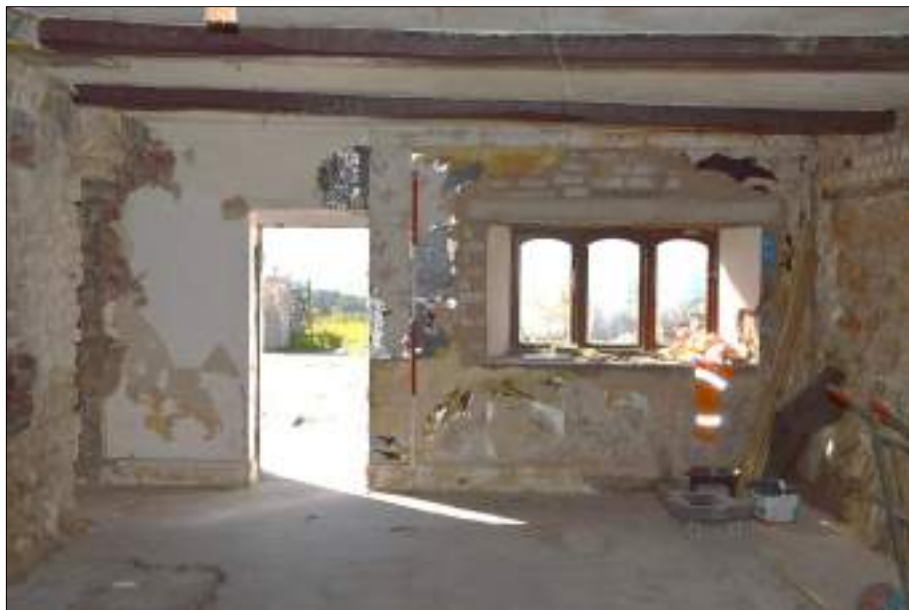
Plate 20 (shot 47): Southeastern wall, Room 1, 2m scale
