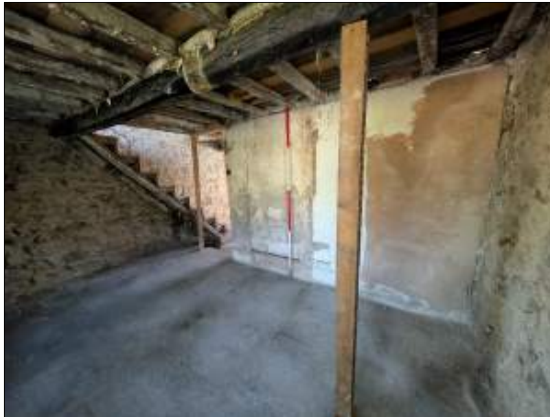
Plate 47 (shot 180): Southwestern wall of Room 3, 2m scale
