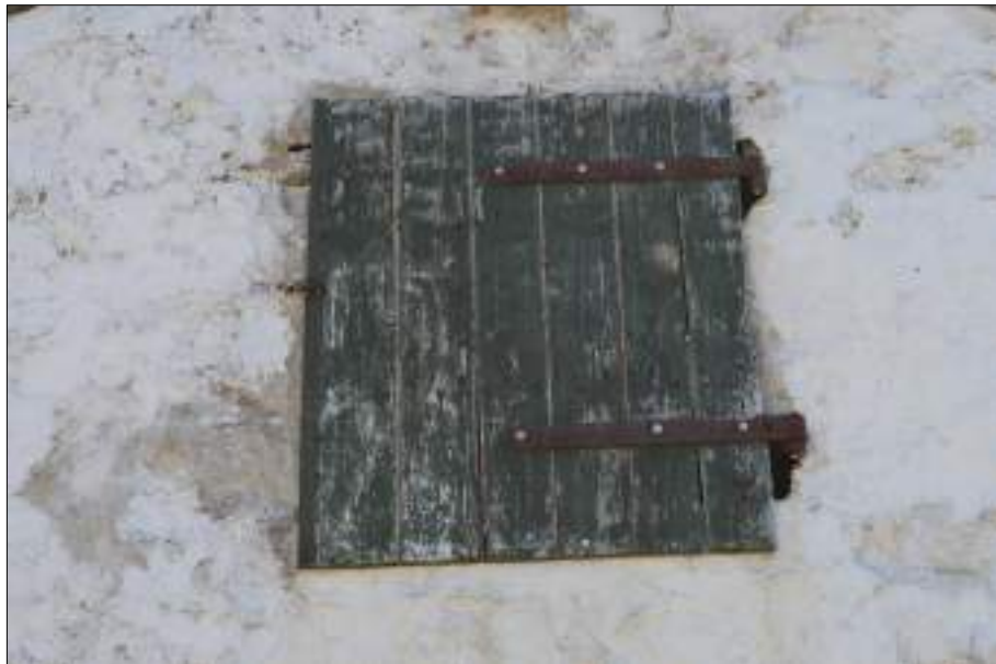
Plate 108 (shot 124): Detail of door in southwestern wall of outbuilding, 2m scale
