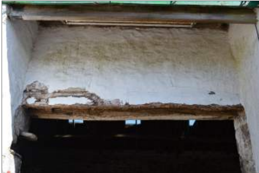
Plate 84 (shot 11): Timber lintel over entranceway, southeast facing elevation of barn, no scale
