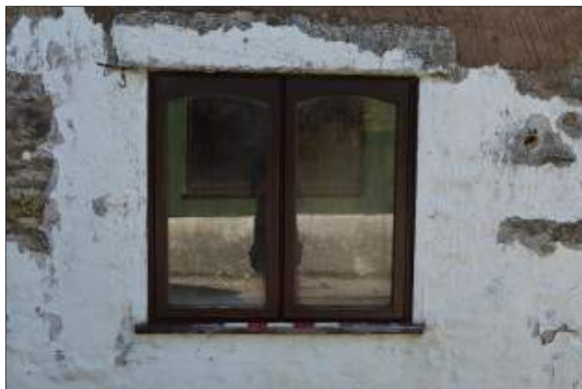
Plate 5 (shot 39): Detail of ground floor window in southwest facing elevation of farmhouse, looking northeast, 0.5m scale
