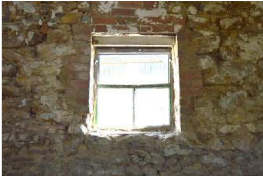
Plate 98 (shot 112): Detail of window, northeast wall of Room 6, 0.5m scale
