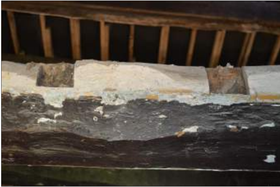
Plate 51 (shot 87): Detail of mortise joints in ceiling beam, Room 4, no scale
