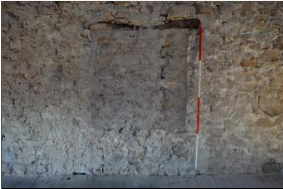
Plate 68 (shot 88): Detail of blocked window, southwestern wall of Room 5, 2m scale
