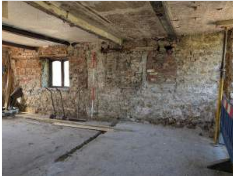
Plate 15 (shot 173): Interior of Room 1, looking southwest, 2m scale
