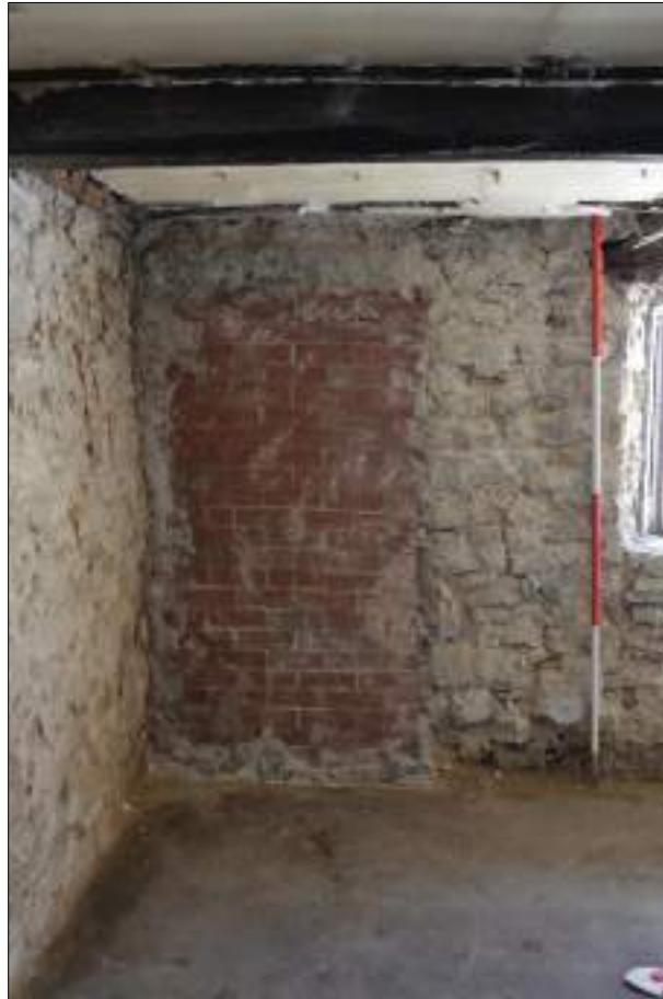
Plate 34 (shot 60): Detail of blocked doorway in southeastern wall of Room 2, 2m scale
