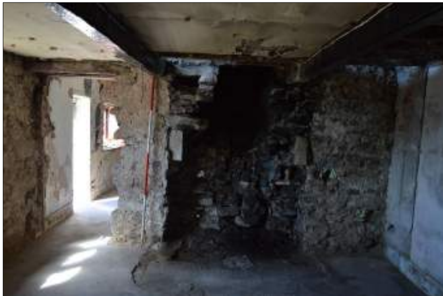
Plate 35 (shot 61): Southwestern wall of Room 2, 2m scale
