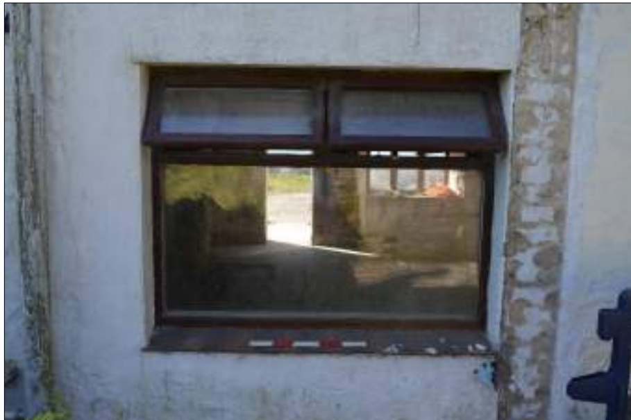
Plate 10 (shot 31): Detail of ground floor window, northwest elevation of farmhouse, 0.5m scale
