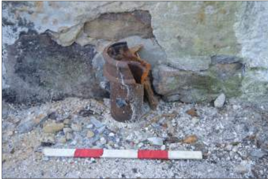
Plate 14 (shot 27): Cast iron pipe on northwestern side of farmhouse, 0.5m scale
