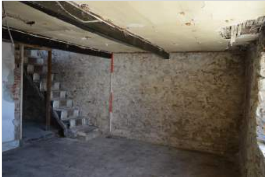
Plate 32 (shot 55): Interior of Room 2, looking northeast, 2m scale
