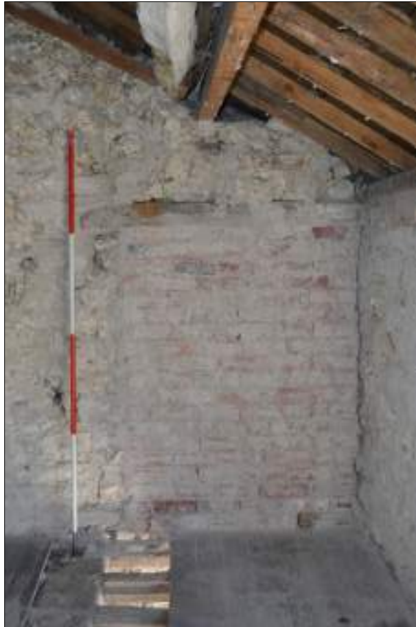
Plate 62 (shot 92): Detail of blocked doorway, northeastern wall of Room 5, 2m scale
