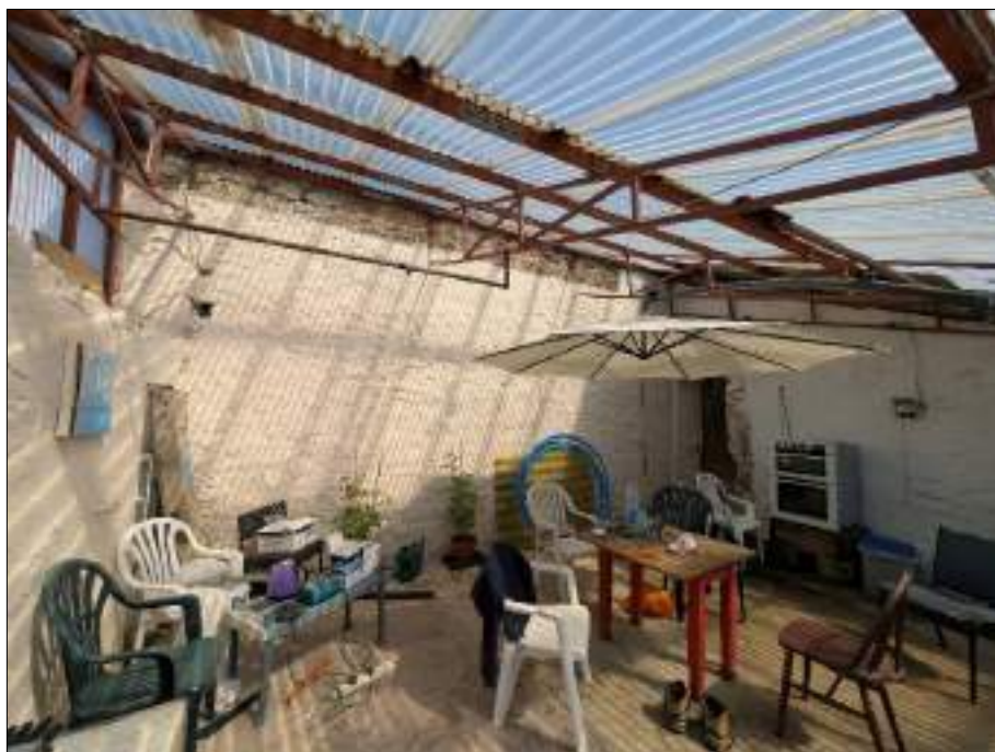
Plate 131 (shot 204): Interior of Room 11, 2m scale
