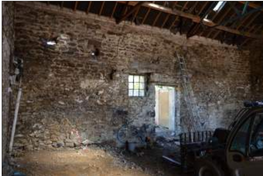
Plate 92 (shot 100): Northwestern wall of Room 6, 2m scale
