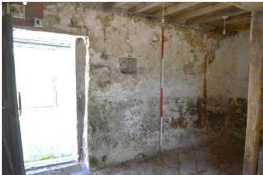
Plate 121 (shot 142): Northwestern wall of Room 7, 2m scale
