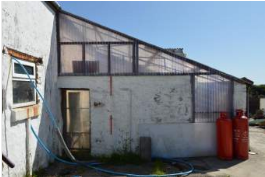
Plate 116 (shot 125): Southwestern elevation of extension to outbuilding, 2m scale
