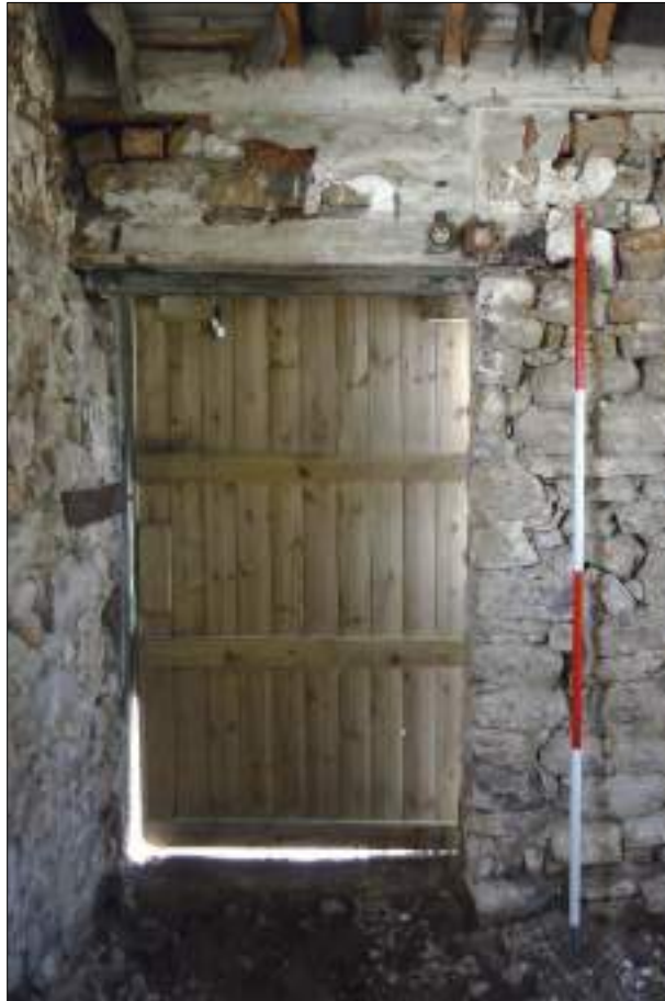
Plate 101 (shot 116): Detail of doorway in southeastern wall of outshut, Room 6, 2m scale
