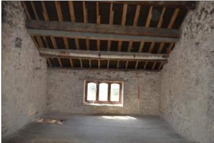
Plate 72 (shot 96): Southeast side of Room 5 showing roof construction, 1m and 0.5m scales
