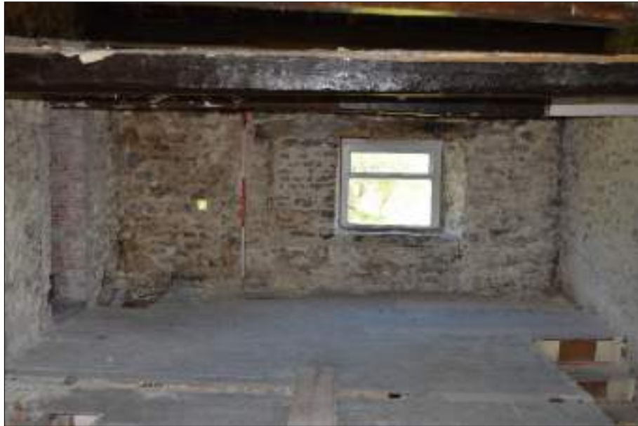
Plate 57 (shot 76): Northwestern wall of Room 4, 2m scale
