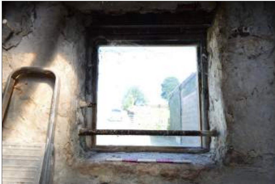
Plate 130 (shot 150): Detail of window in northwestern wall of Room 8, 0.5m scale
