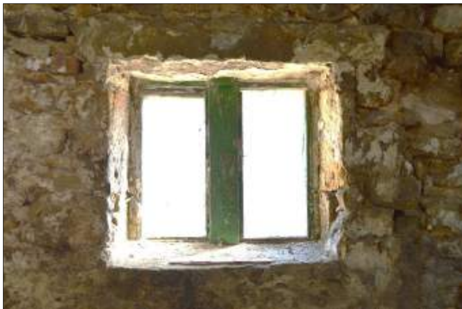
Plate 97 (shot 111): Detail of window, northeast wall of Room 6, 0.5m scale
