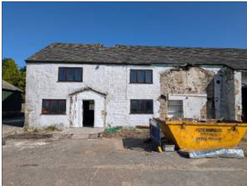
Plate 1 (shot 166): Southeast-facing elevation of farmhouse, looking northwest, 2m scale
