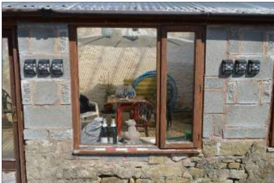
Plate 119 (shot 132): Detail of window in southeastern elevation of extension to outbuilding, 0.5m scale
