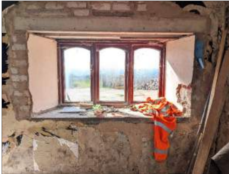
Plate 21 (shot 175): Detail of window, southeastern wall, Room 1, 0.5m scale
