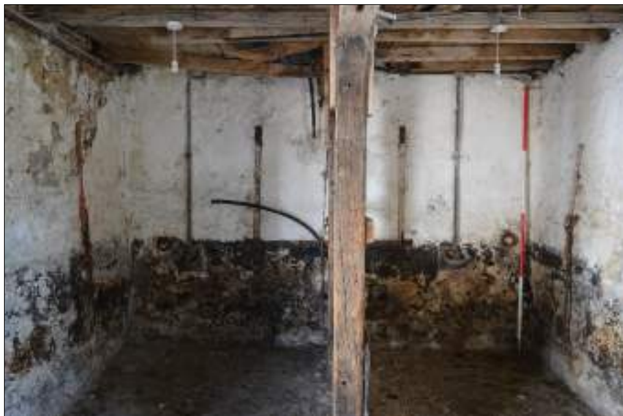
Plate 123 (shot 140): Northeastern wall of Room 7, 2m scale
