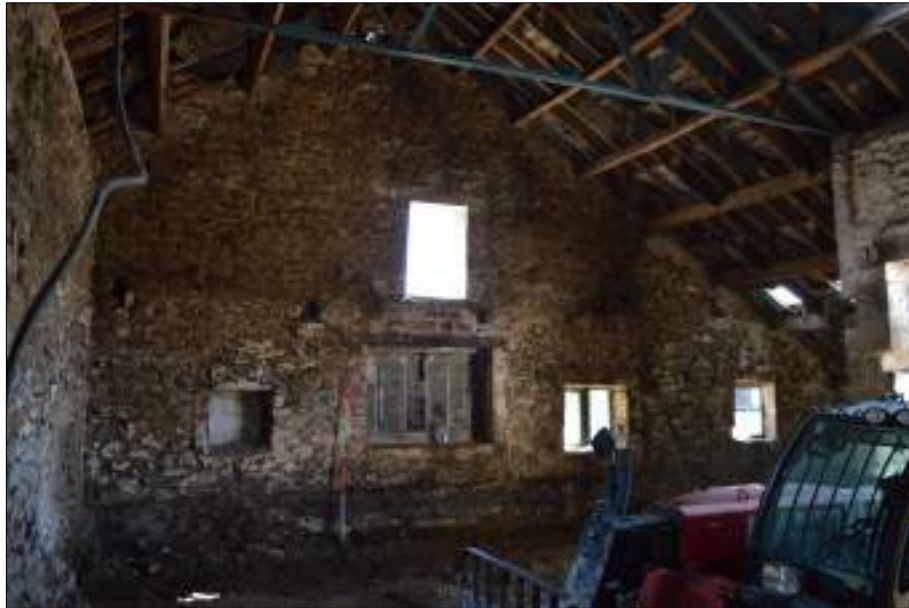
Plate 94 (shot 107): Northeastern wall of Room 6, 2m scale
