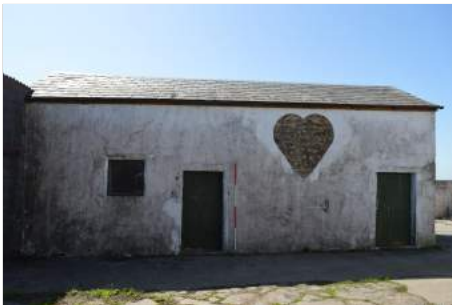
Plate 109 (shot 133): Northwestern elevation of outbuilding, 2m scale
