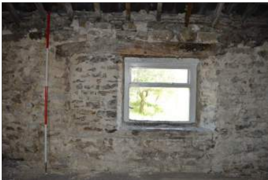
Plate 58 (shot 78): Detail of window, northwestern wall of Room 4, 2m and 0.5m scales
