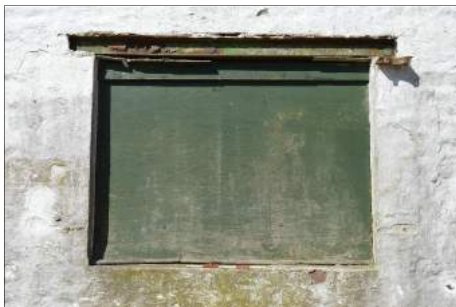
Plate 77 (shot 19): Detail of window in northeast elevation of barn, 0.5m scale
