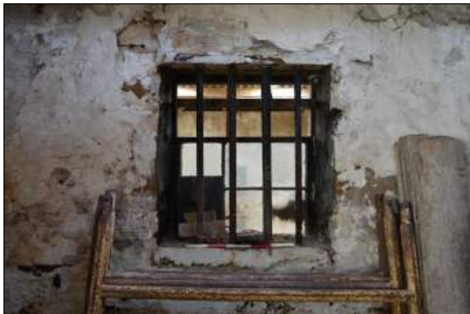
Plate 129 (shot 147): Detail of window in northeastern wall of Room 8, 0.5m scale
