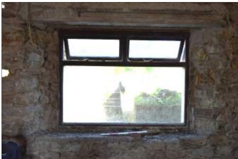
Plate 30 (shot 42): Detail of window, northwestern wall, Room 1, 0.5m scale
