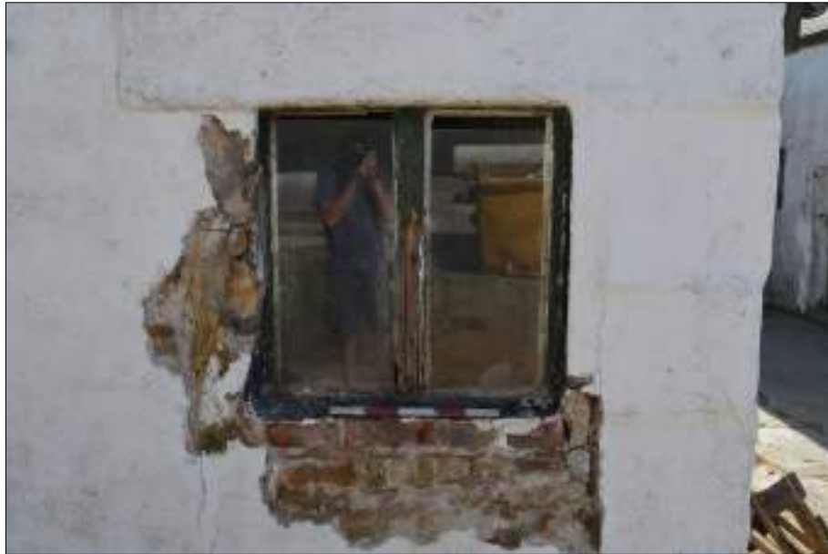
Plate 88 (shot 5): Detail of window, southwest elevation of outshut, 0.5m scale
