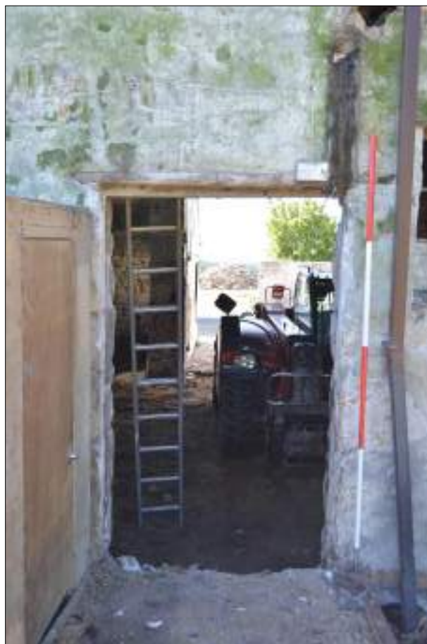
Plate 75 (shot 25): Detail of doorway in northwest elevation of barn, 2m scale
