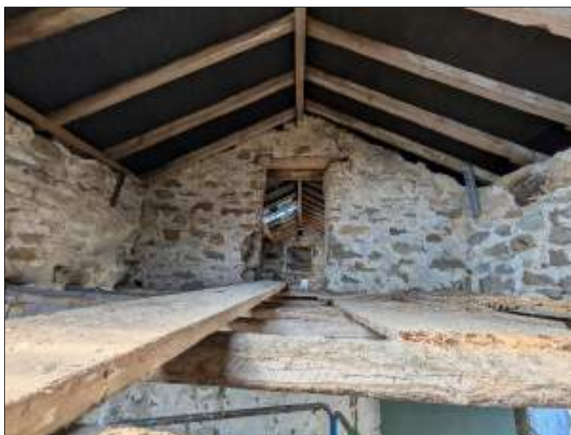
Plate 134 (shot 199): Southwestern wall of Room 10, no scale
