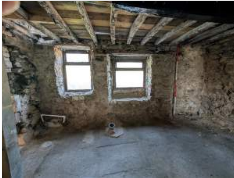
Plate 43 (shot 181): Northwestern wall of Room 3, 2m scale
