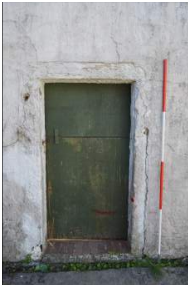
Plate 112 (shot 134): Detail of door in northwestern elevation of outbuilding, 2m scale
