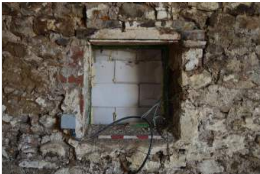
Plate 95 (shot 108): Detail of window, northeast wall of Room 6, 0.5m scale
