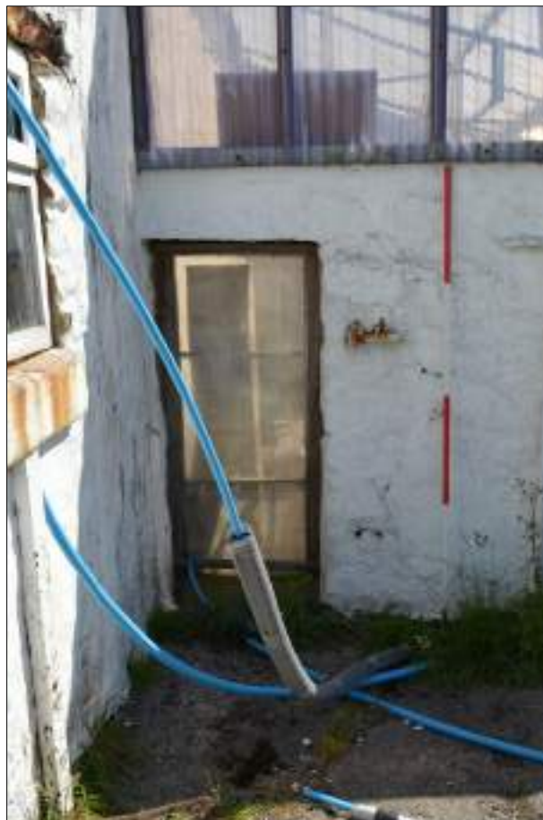
Plate 117 (shot 126): Detail of door in southwestern elevation of extension to outbuilding, 2m scale
