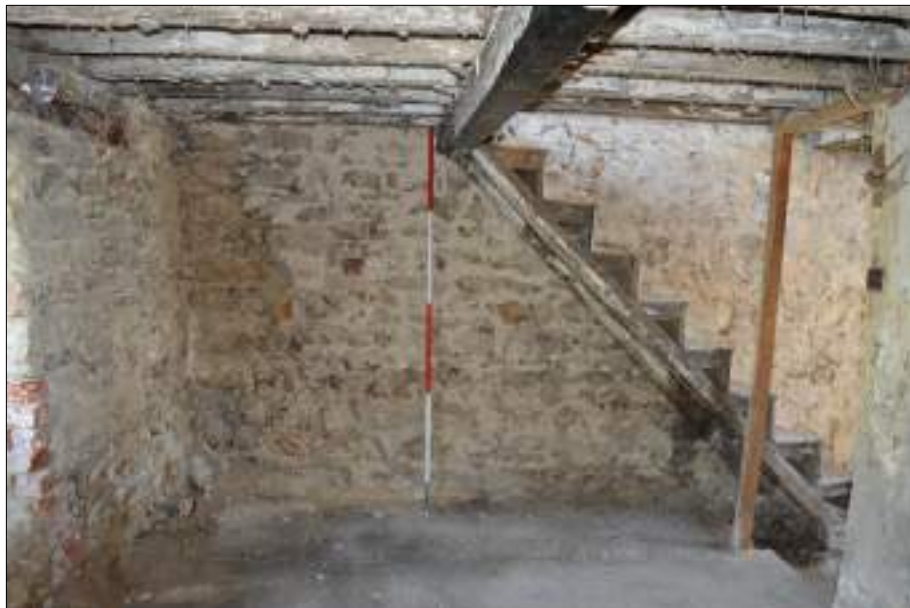
Plate 40 (shot 69): Northeastern wall of Room 2, 2m scale
