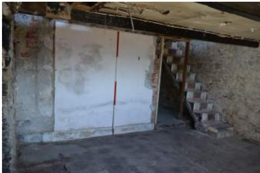
Plate 37 (shot 65): Northwestern wall of Room 2, 2m scale
