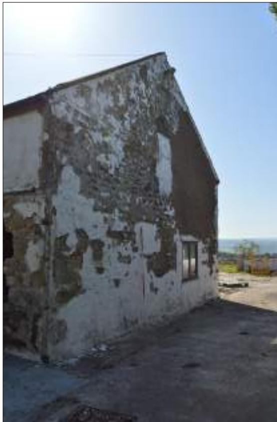
Plate 4 (shot 36): Southwest-facing elevation of farmhouse, looking southeast, 2m scale
