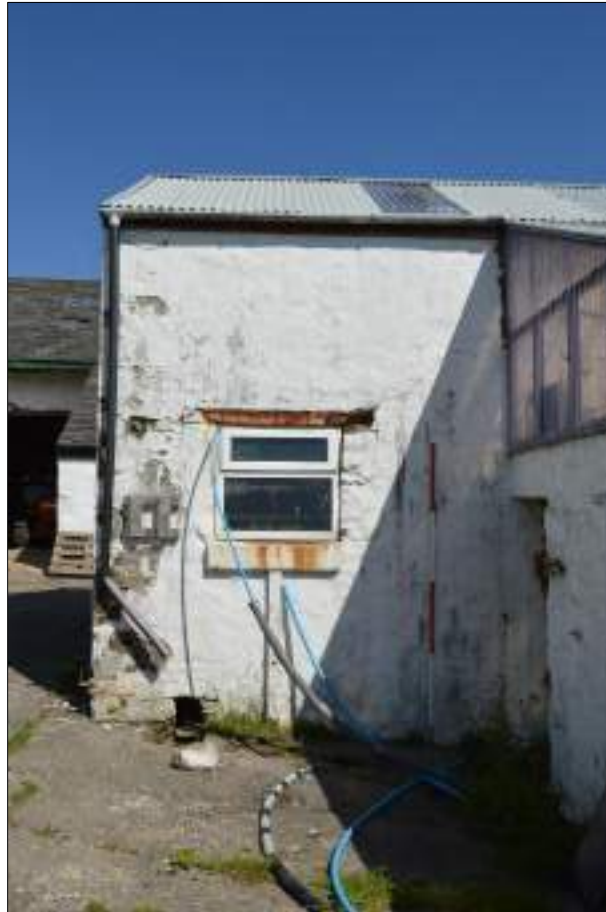
Plate 114 (shot 127): Southeastern elevation of outbuilding, southwestern end, 2m scale
