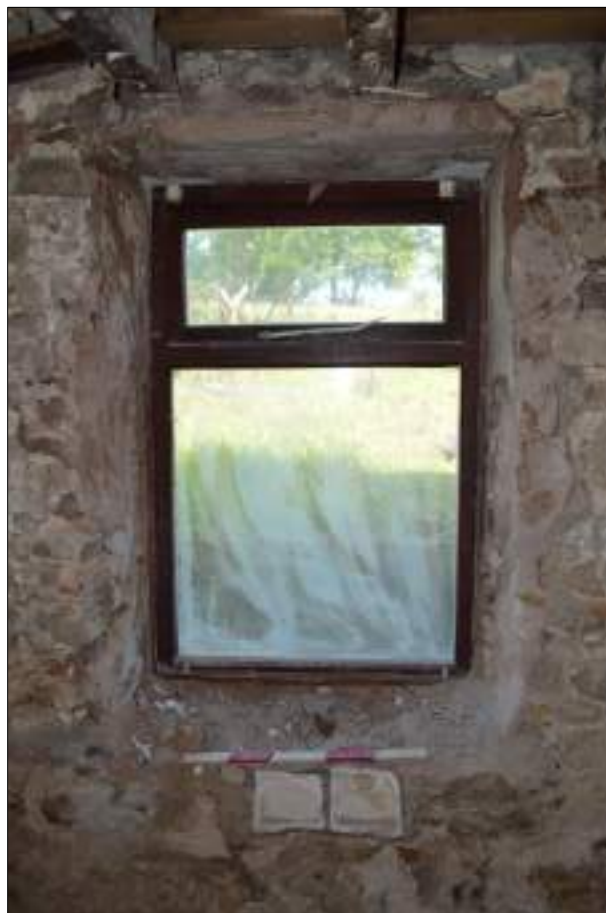
Plate 44 (shot 73): Detail of window, northwestern wall, Room 3, 0.5m scale
