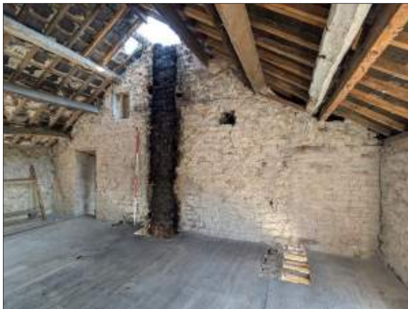
Plate 60 (shot 189): Interior of Room 5, looking northeast, 2m scale
