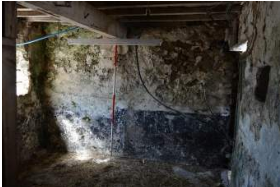
Plate 120 (shot 144): Southwest wall of Room 7, 2m scale
