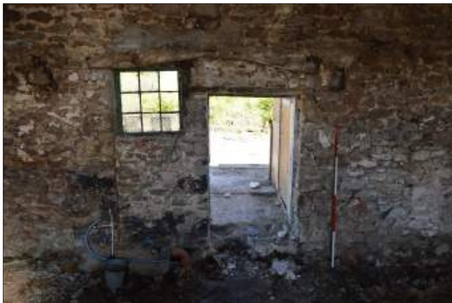
Plate 93 (shot 102): Remodelled entranceway in northwestern wall of Room 6, 2m scale
