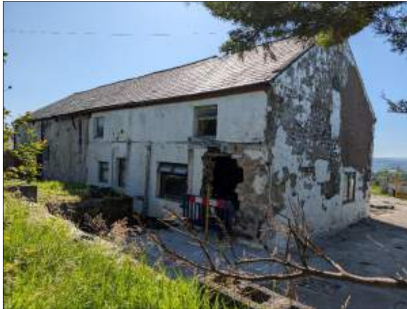
Plate 7 (shot 172): Northwest-facing elevation of farmhouse, looking southeast, 2m scale
