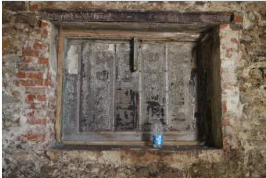
Plate 96 (shot 109): Detail of window, northeast wall of Room 6, 0.5m scale
