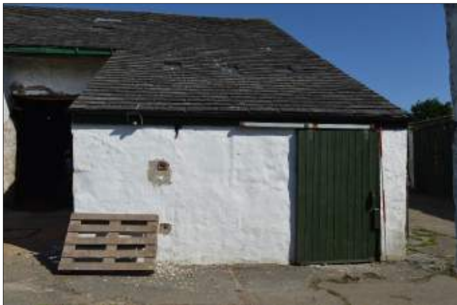
Plate 85 (shot 13): Southeast-facing elevation of outshut, northeast end of main range, 2m scale
