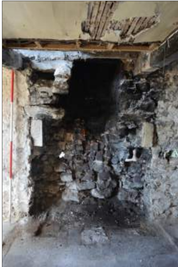
Plate 36 (shot 62): Detail of demolished fireplace, southwestern wall of Room 2, 2m scale
