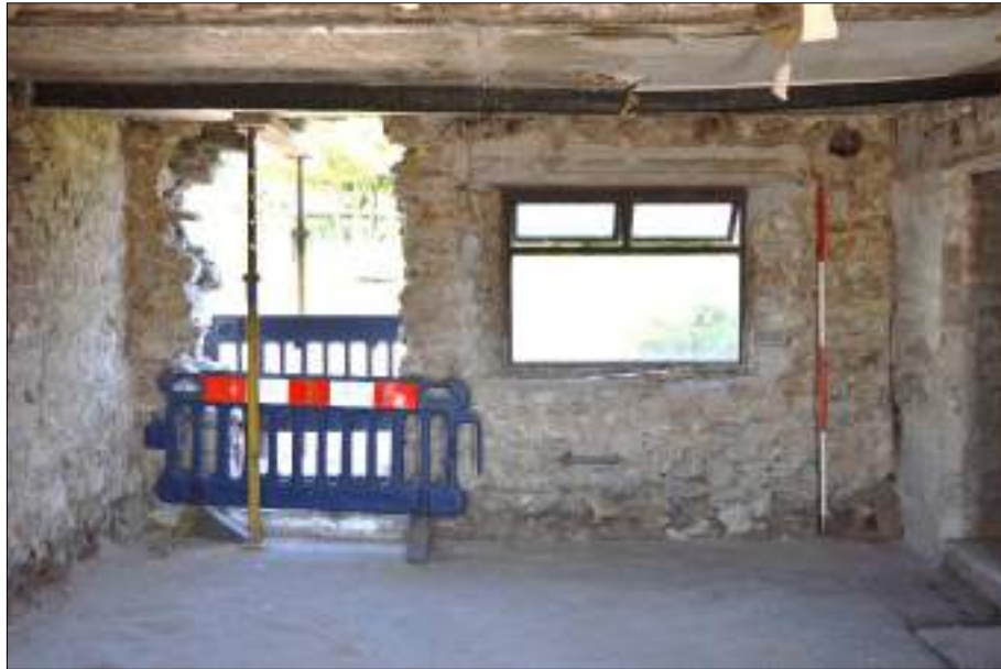
Plate 29 (shot 41): Northwestern wall, Room 1, 2m scale
