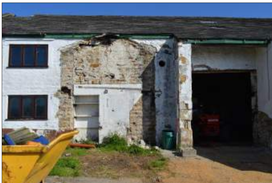
Plate 82 (shot 1): Southeast facing elevation of barn, southwest end, 2m scale
