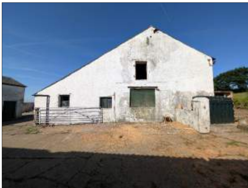
Plate 76 (shot 171): Northeast facing elevation of barn, 2m scale
