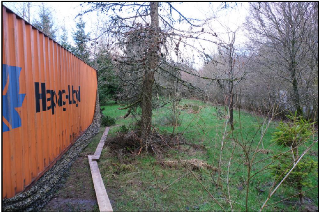
Image showing metal container (proposed toilet block) along the north boundary of the development site
