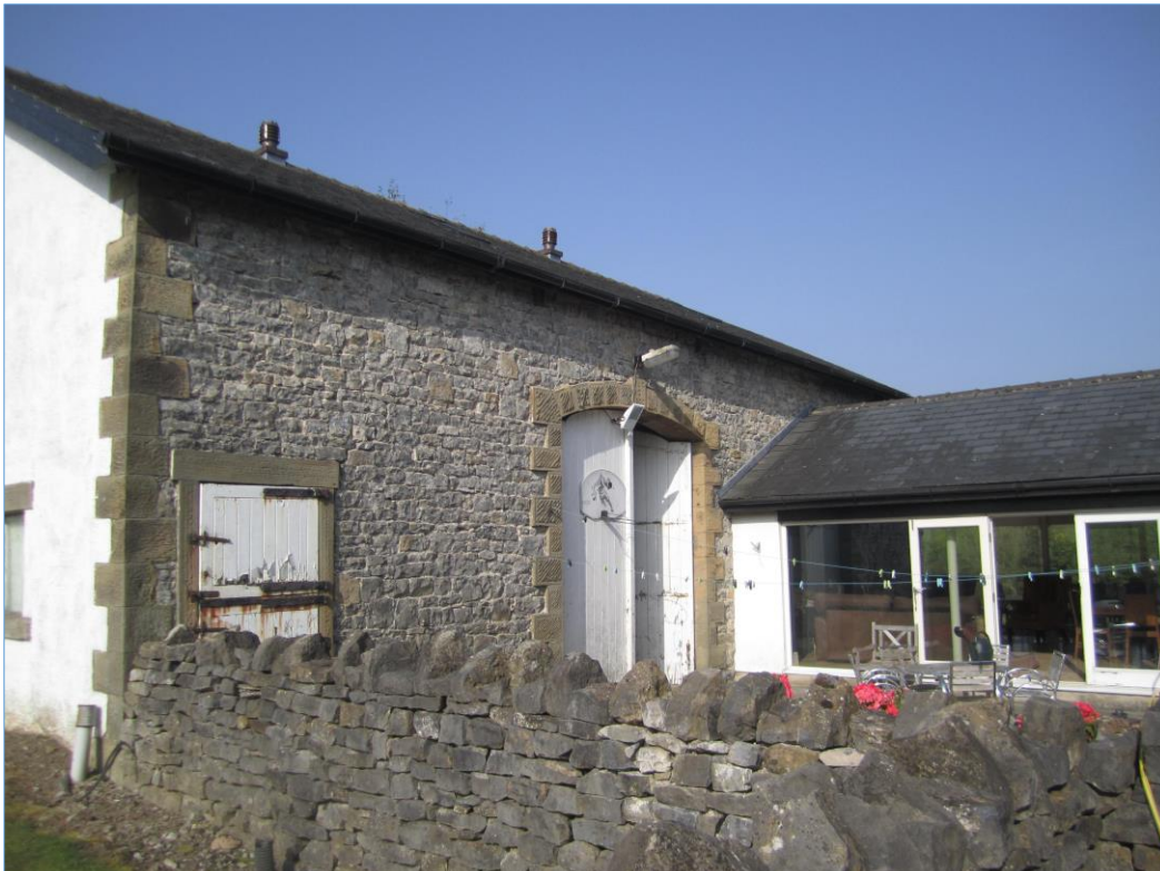
1 Northeast elevation of the barn
