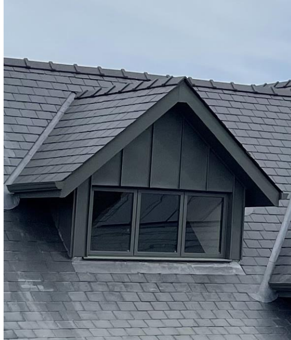
Pl. 2 Example of a dormer roof window
