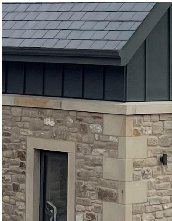
Pl. 7 Photograph showing zinc cladding in conjunction with stone and slate
