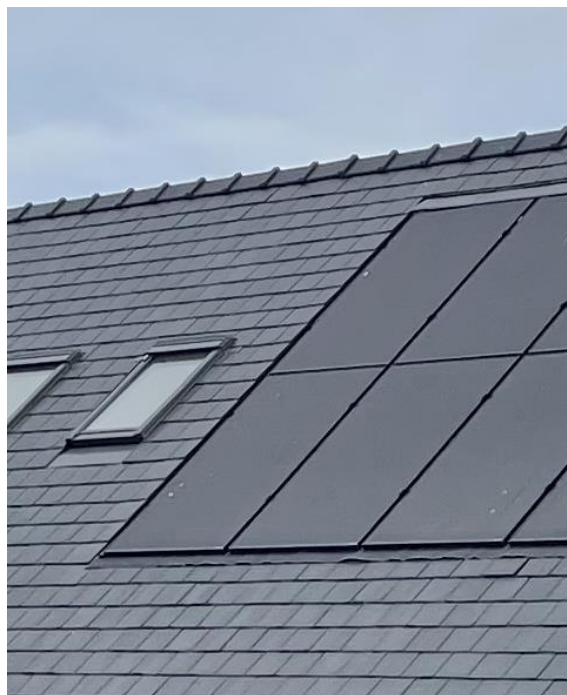
Pl. 1 Photograph showing an example of a new Spanish Blue slate roof with recessed Velux rooflights and black- framed recessed PV solar panels
