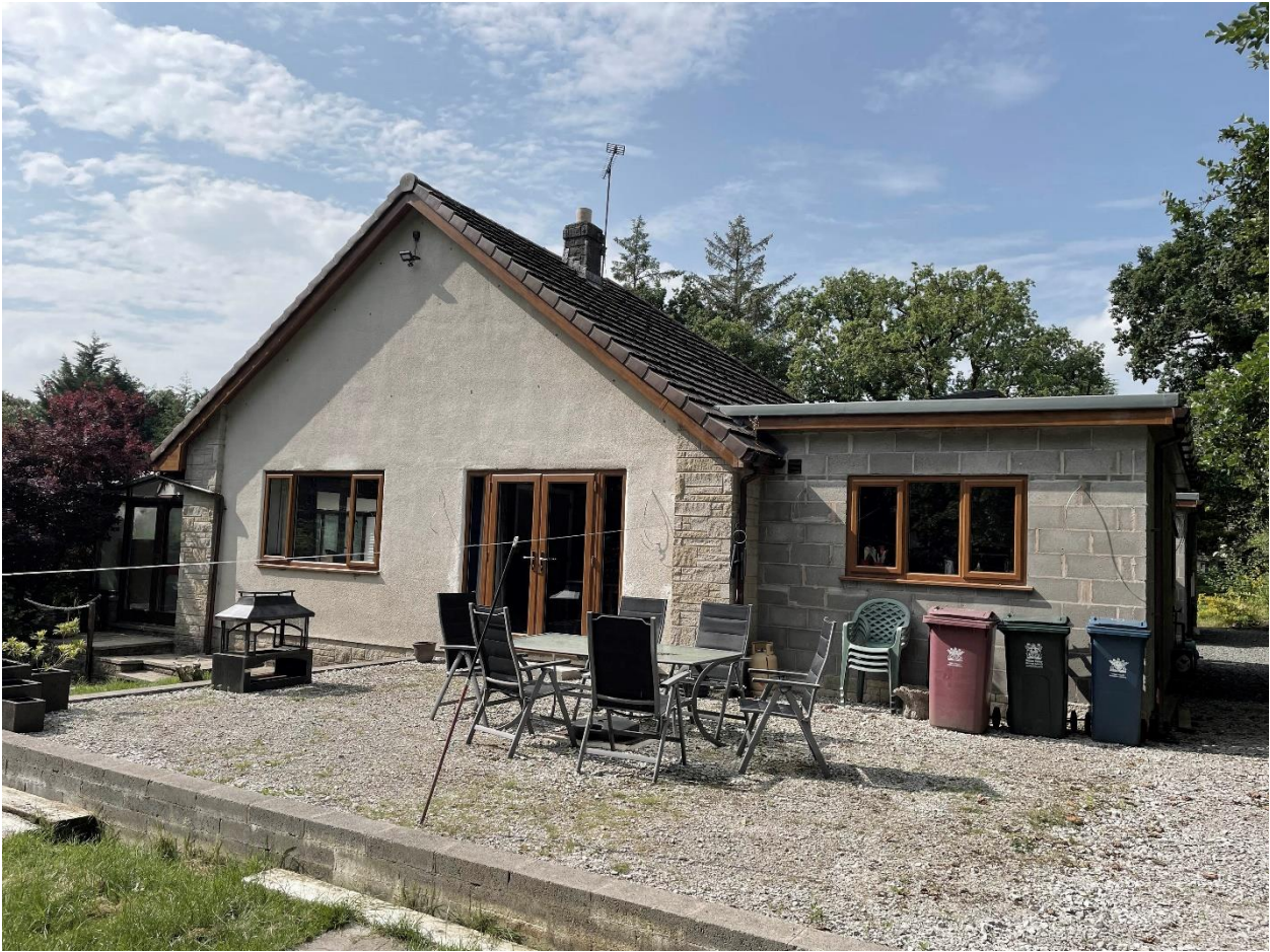
PL03: View of the rear north east facing elevation of the building.
