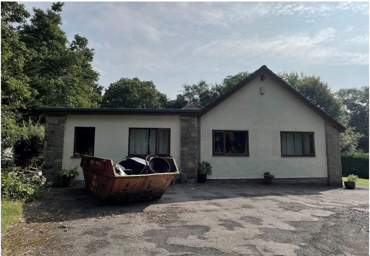
PL02: View of the front south west facing elevation of the building.
