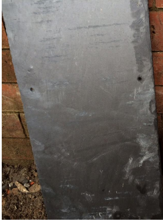
Pl. 1 Photograph showing new Spanish Blue Sumo Best (20x10”) slate for roofs
