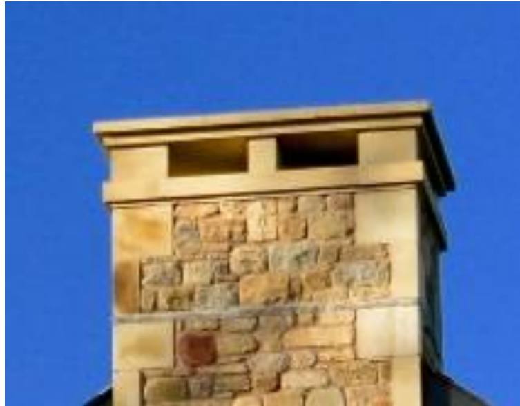
Pl. 5 Photo showing an example of the chimney detail showing the proposed dressed natural stone for window/ door surrounds, quoins, chimney capping and string course. This also shows the proposed reclaimed natural stone for the chimney and external house and garden walls, to be laid to random courses as shown.
