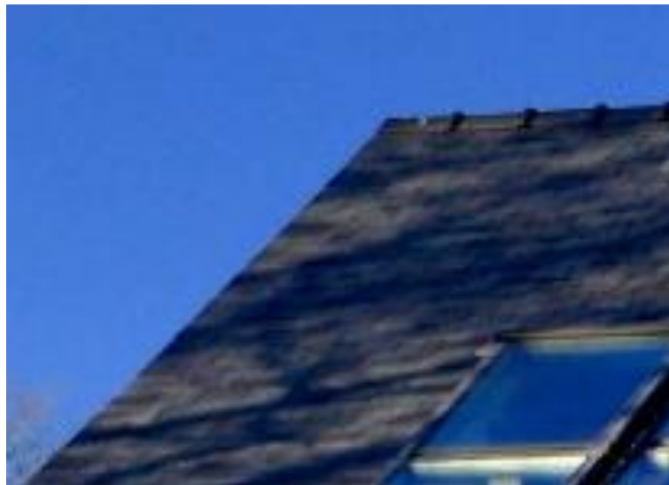
Pl. 2 Photograph showing an example of a new Spanish Blue Sumo Best (20x10”) slate roof with flush fitting Velux rooflight constructed within the Ribble Valley.
