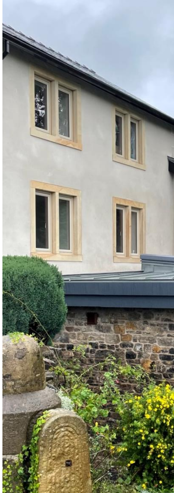
Pl. 7 Photo showing part of a previous project within the Ribble Valley that used the Grey coloured K Rend scraped texture render for external wall finish, with dressed stone surrounds and reclaimed stone walls below
