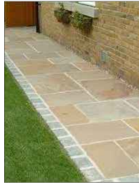
Sandstone flag paving with sett edging
