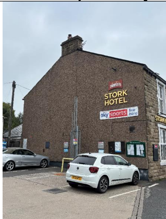
Photograph 4: View of the west facing elevation.
