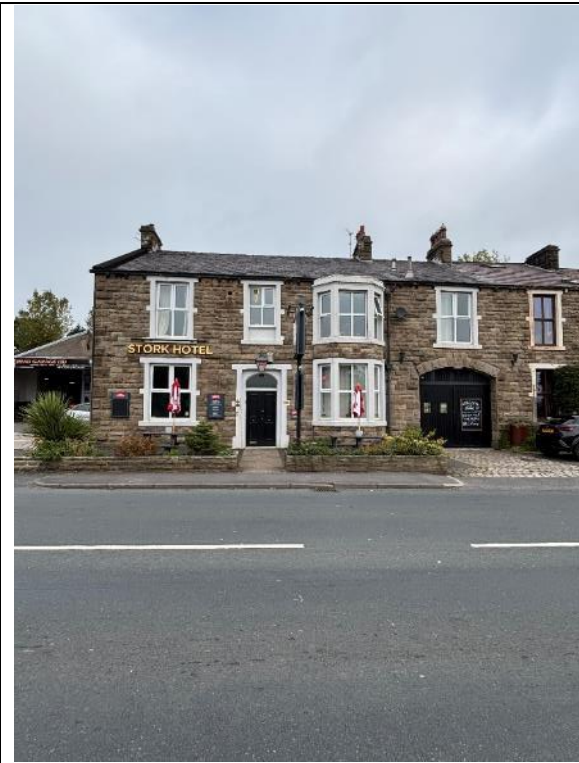
Photograph 1: View of the front of the building (south facing elevation).
