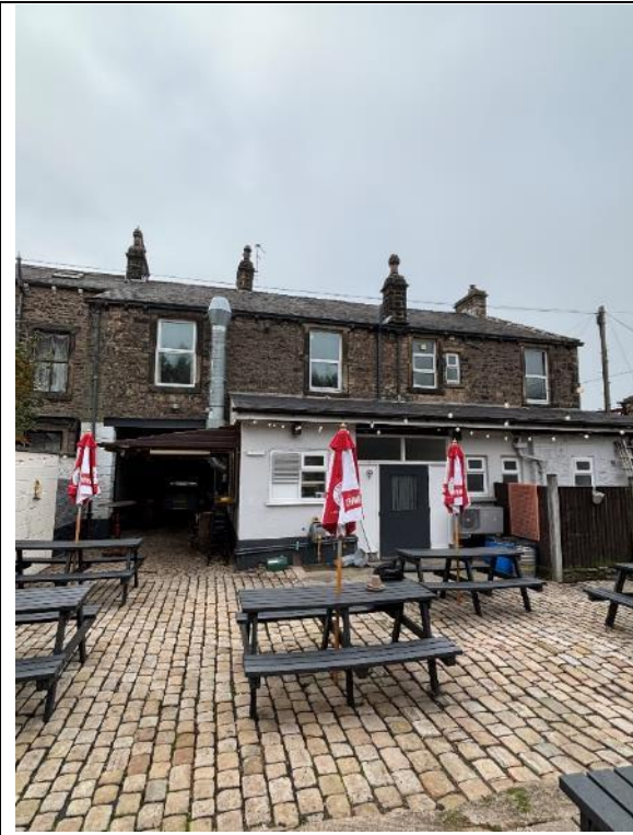
Photograph 5: View north facing elevation.
