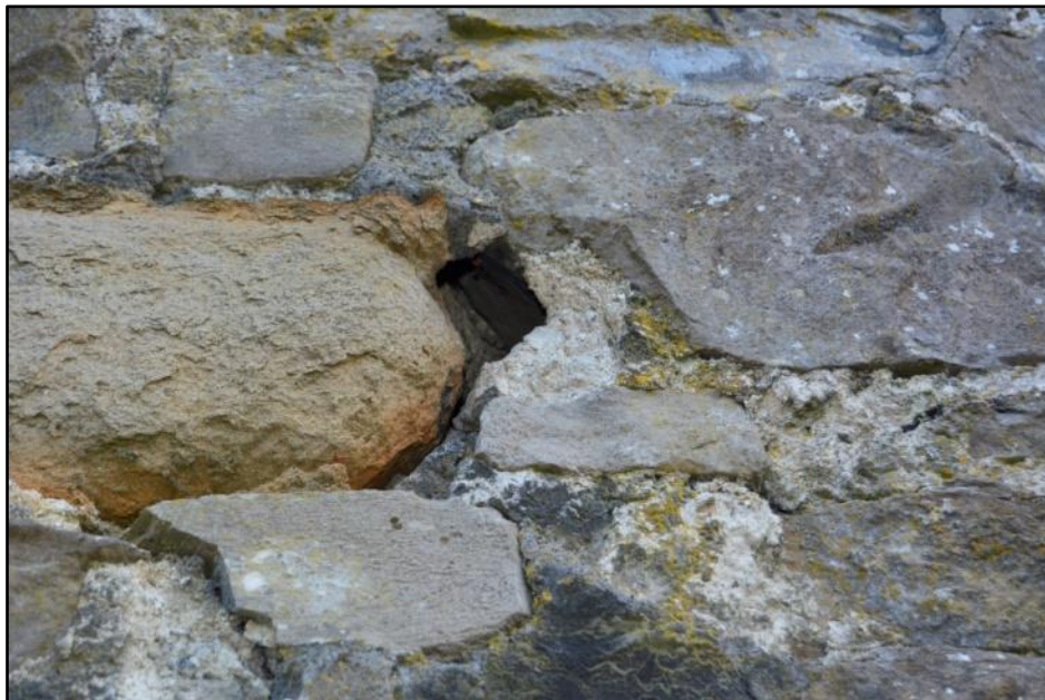
Example of external wall cavity.
