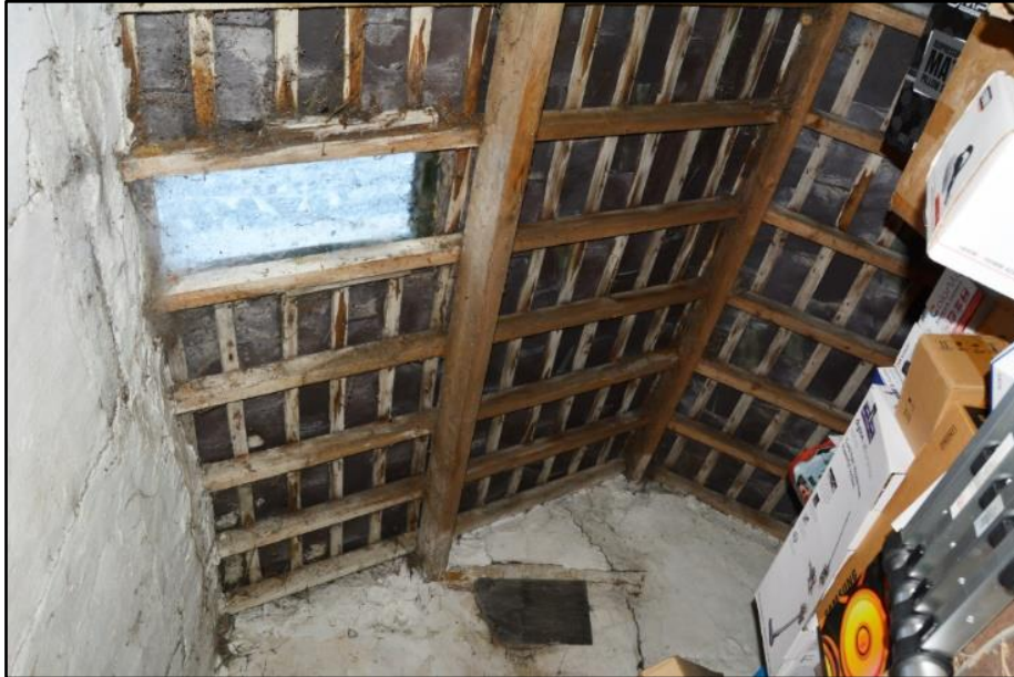
Example of intact roof underside with roof lights. This example is typical of roof underside in all of the buildings. Lack of roof liner in this type of building reduces the likelihood of use by day roosting and hibernating bats.
