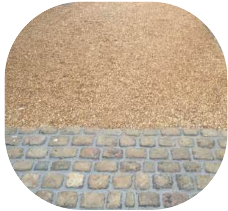
01 Permeable driveway surfacing
