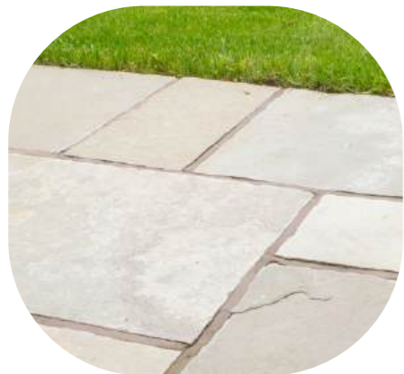
03 Stone paving patios with soft landscaping
