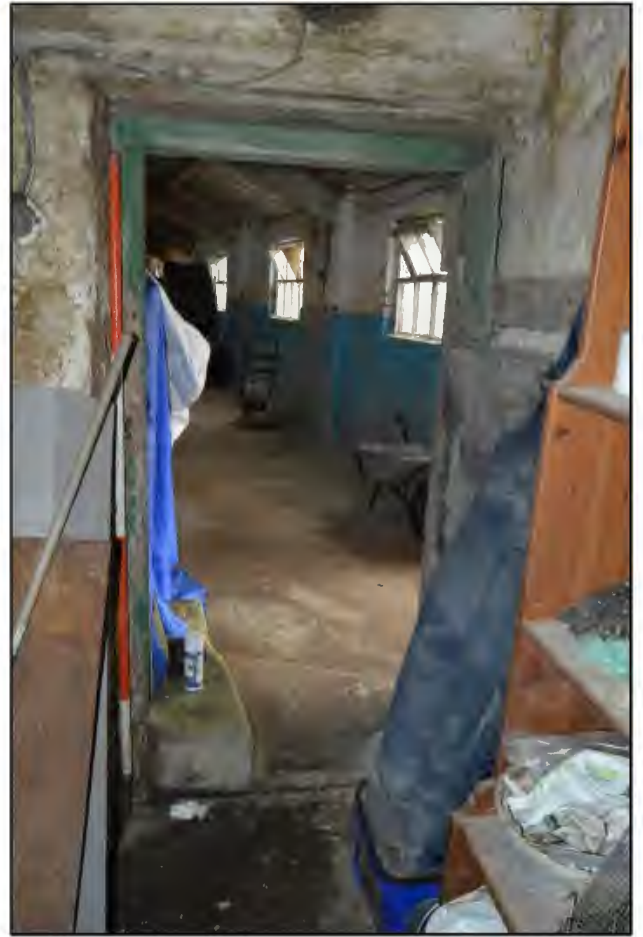
PL53 (right): View south east within store 03 [GF-07].
