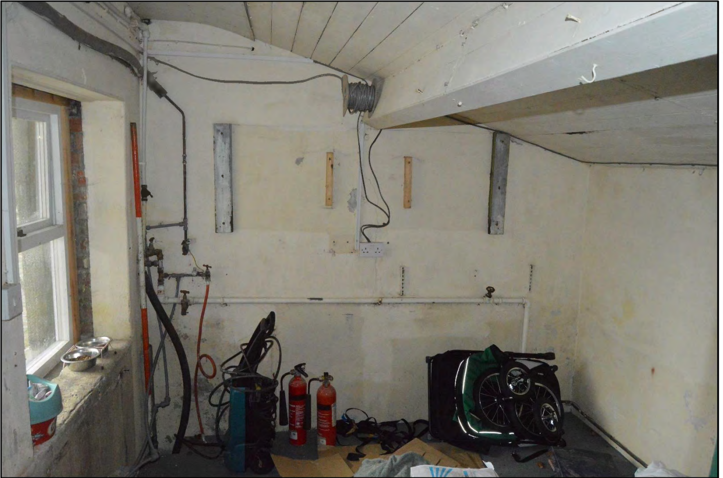
PL60: View north west within the wash house [GF-1 I].
