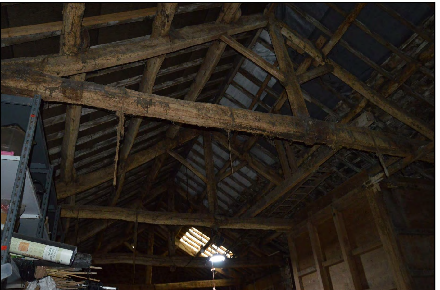
PL39: View of the timber king post roof trusses and associated roof structure over the north end of the barn core.
