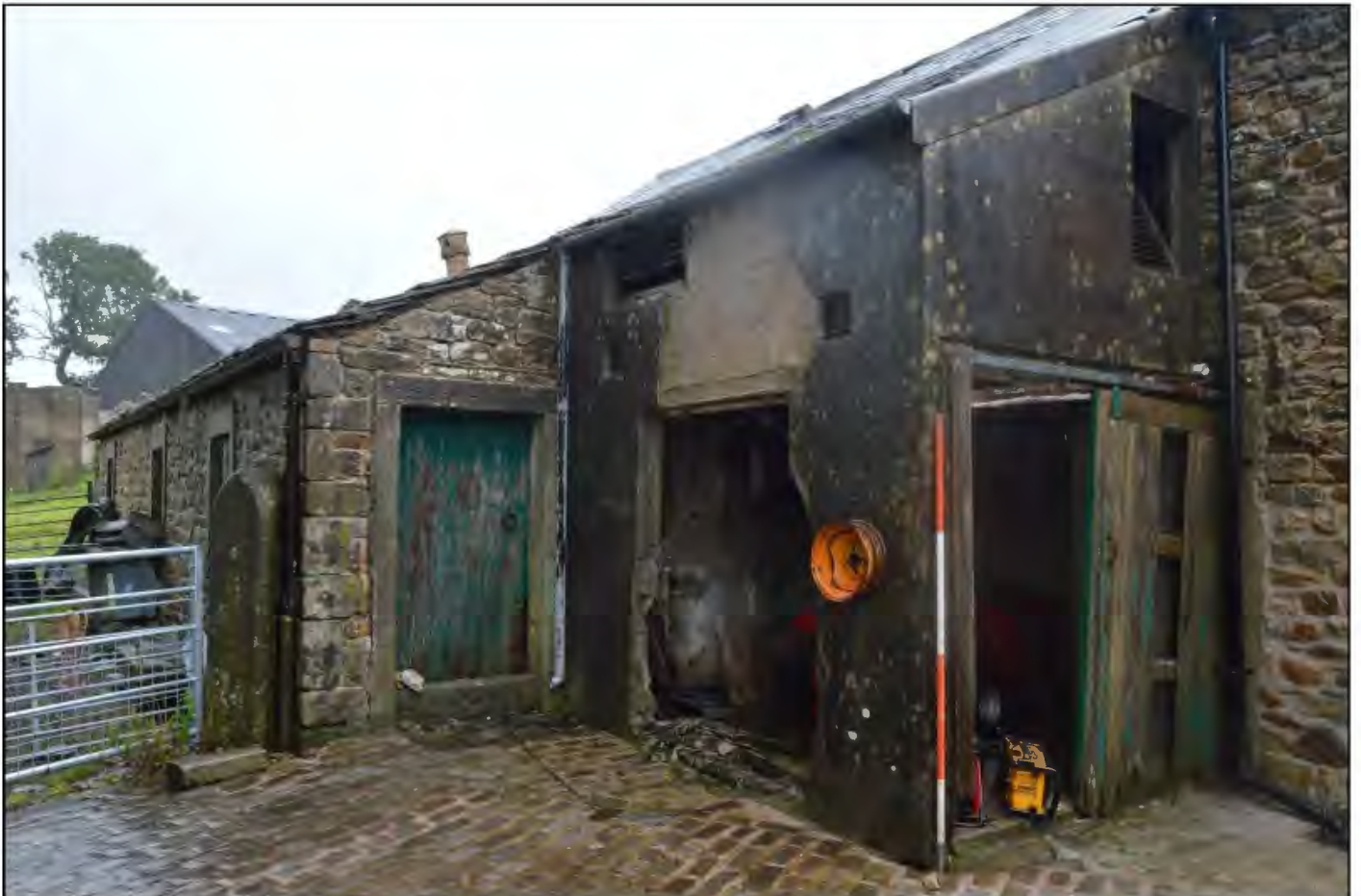
PL16 View of the north west elevation from the south west.
