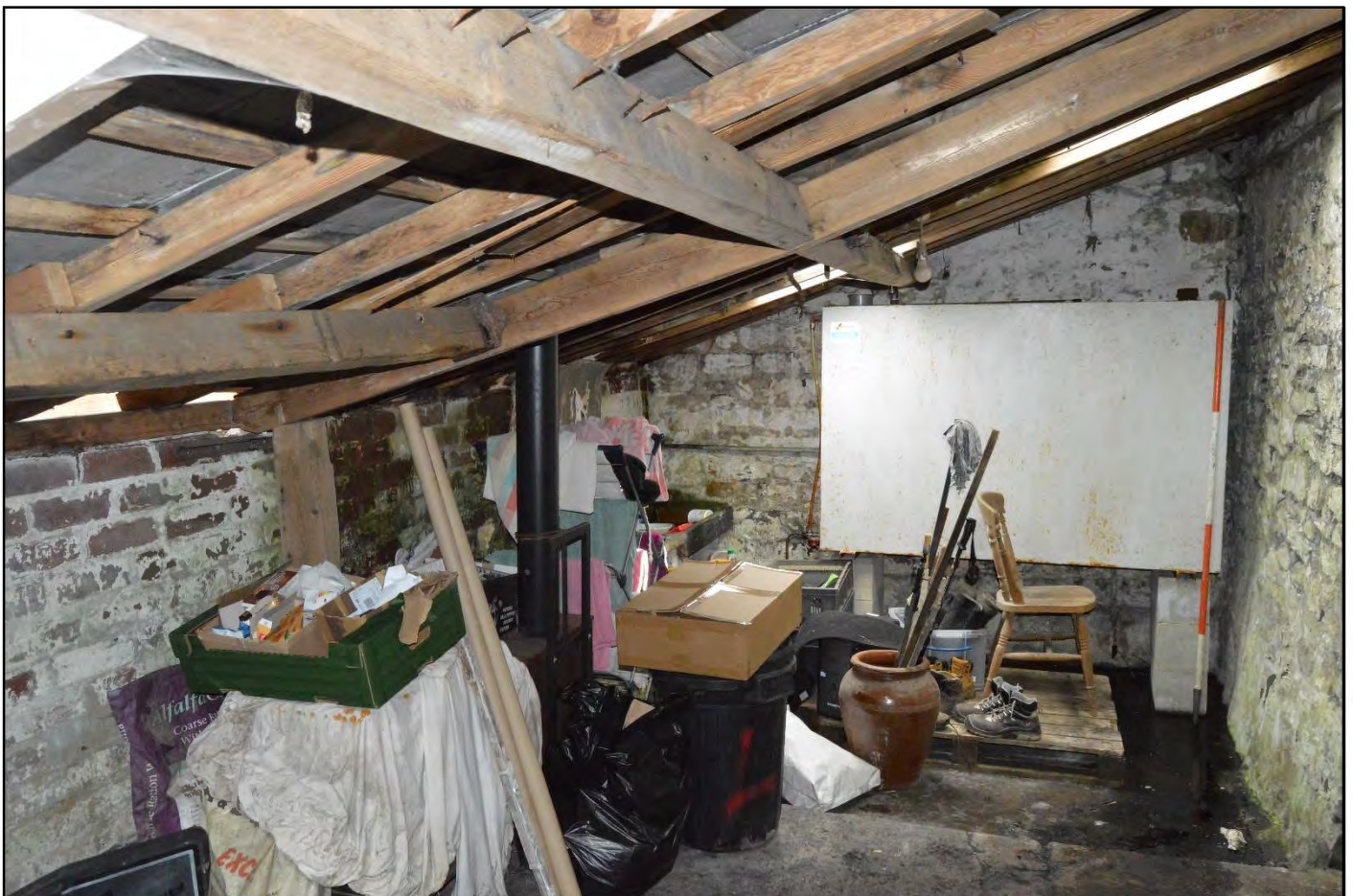
PL63: View south east within the coal store [GF-10].
