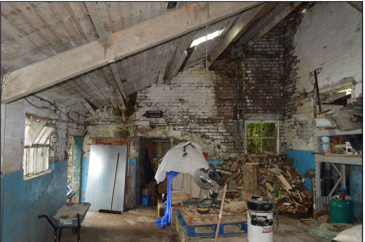
PL69: View west within the former milking parlour [GF-08].
