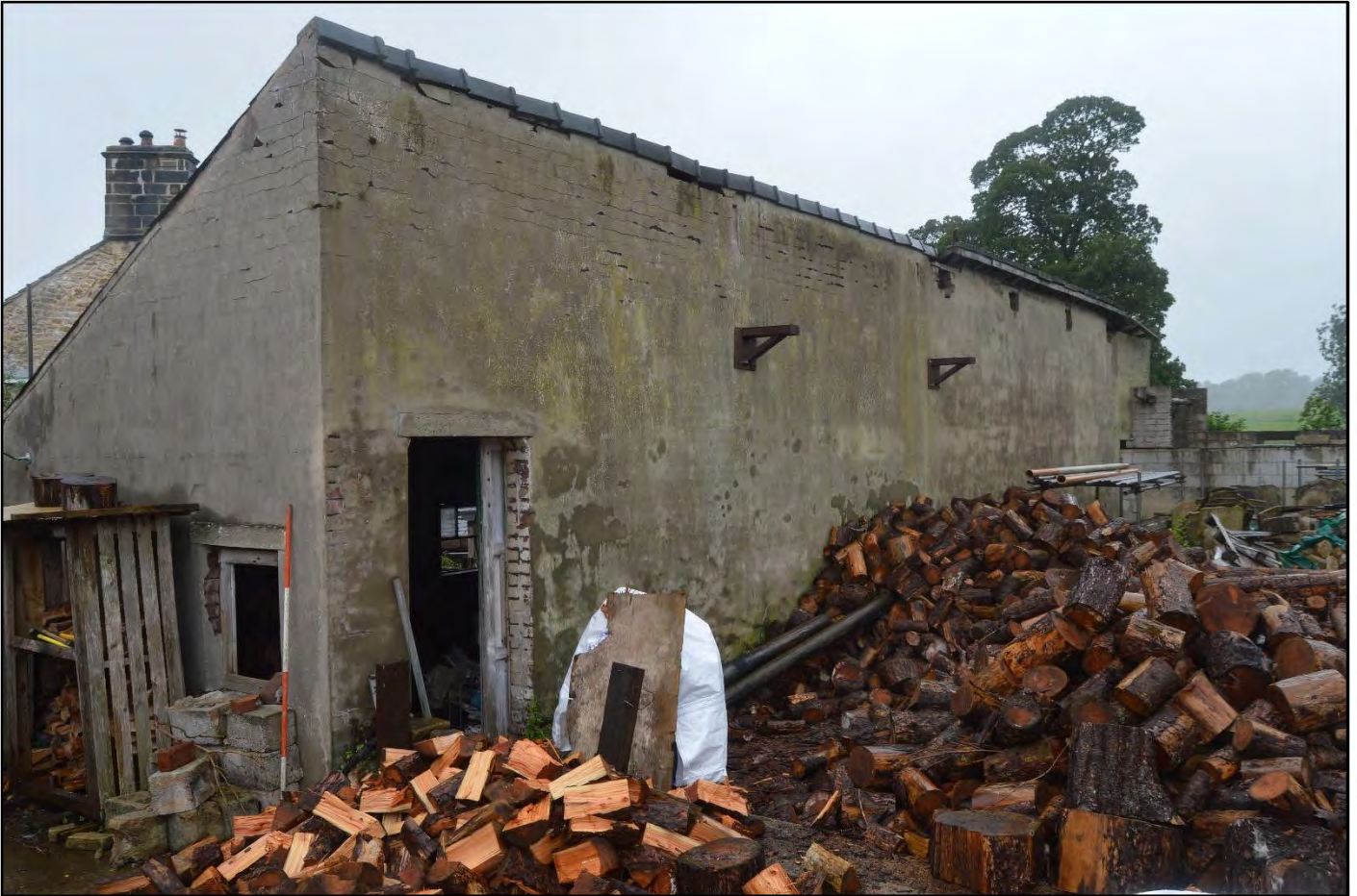
PL68: View of the north elevation of the former milking parlour [GF-08] and wood store [GF-09].
