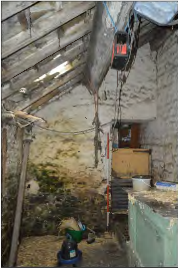
PL49 (left): View south east within store 02 [GF-06].
