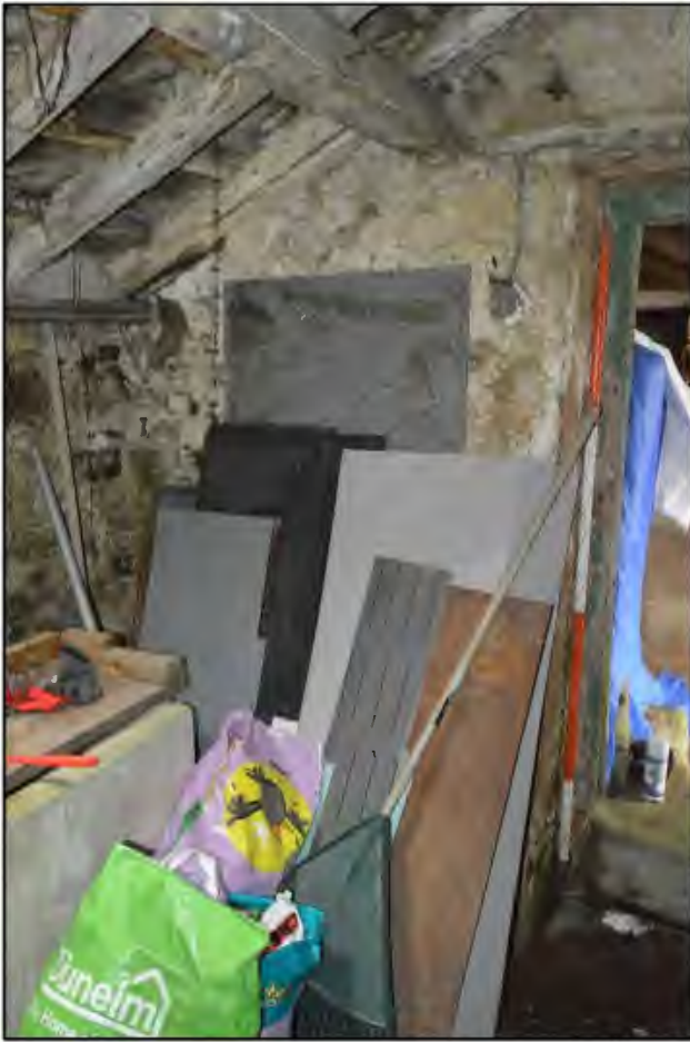
PL52 (left): View south east within store 03 [GF-07].
