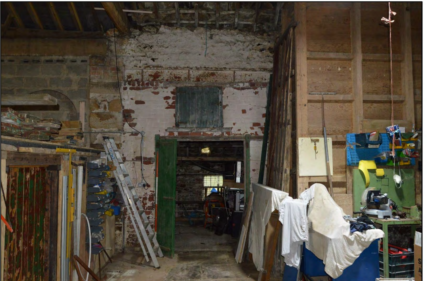
PL29: View north west of infill brickwork opposite the south east cart entry doors [GF-04].
