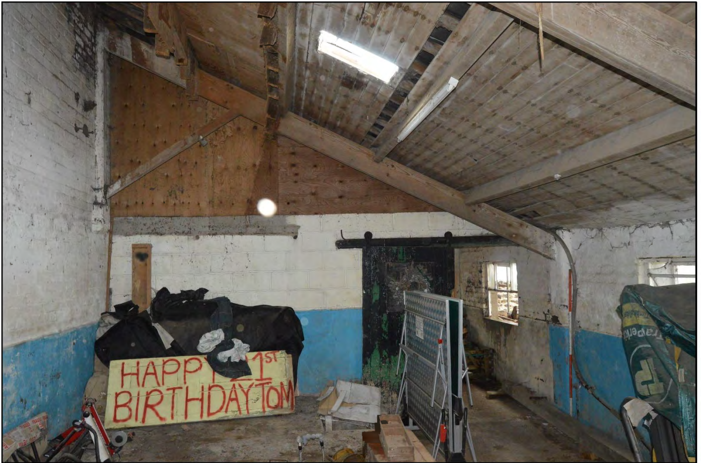
PL72: View east within the former milking parlour [GF-08].
