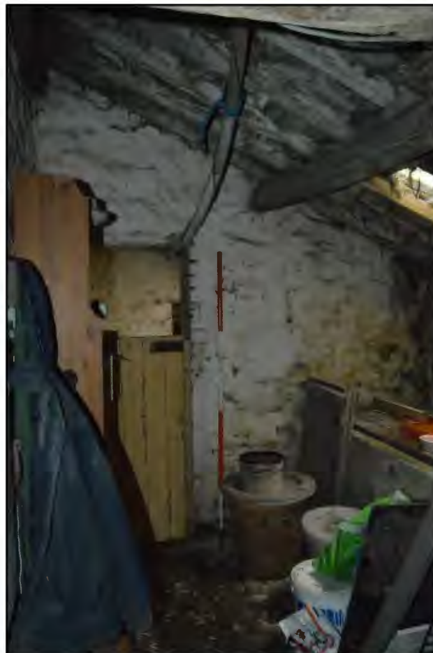
PL51: View North west within store 03 [GF-07].
