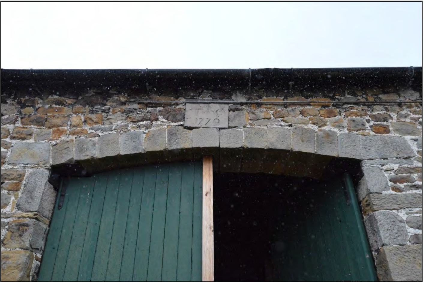
PL03: View of the segmental stone head over the cart entry doors to the south east elevation of the barn.
