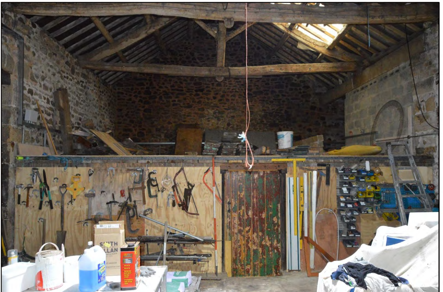
PL33: View south west within the barn, towards the shippon [GF-01] and hay loft [FF-01].
