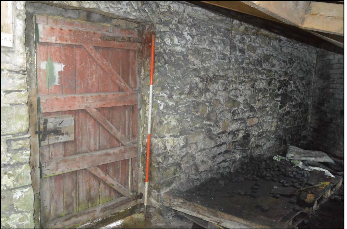
PL64: View west within the coal store [GF-10].
