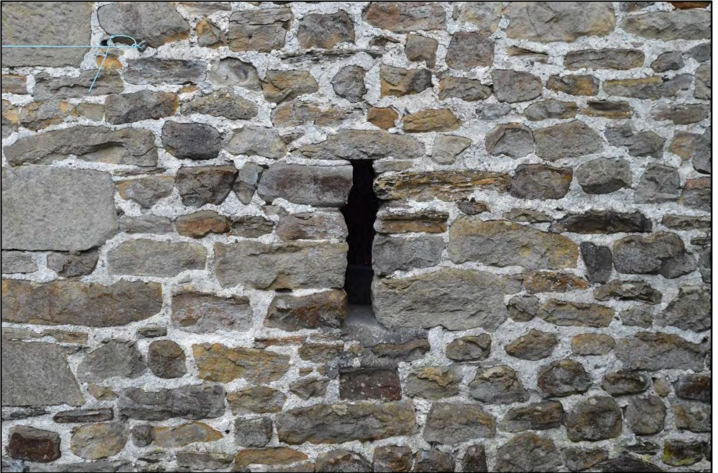
PL05: View of breather detail to the south east elevation of the barn.
