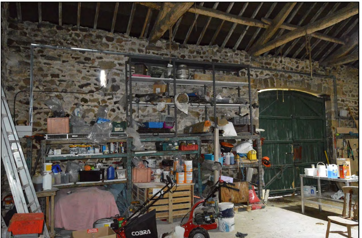
PL31: View south east within the former hay mew [GF-05].
