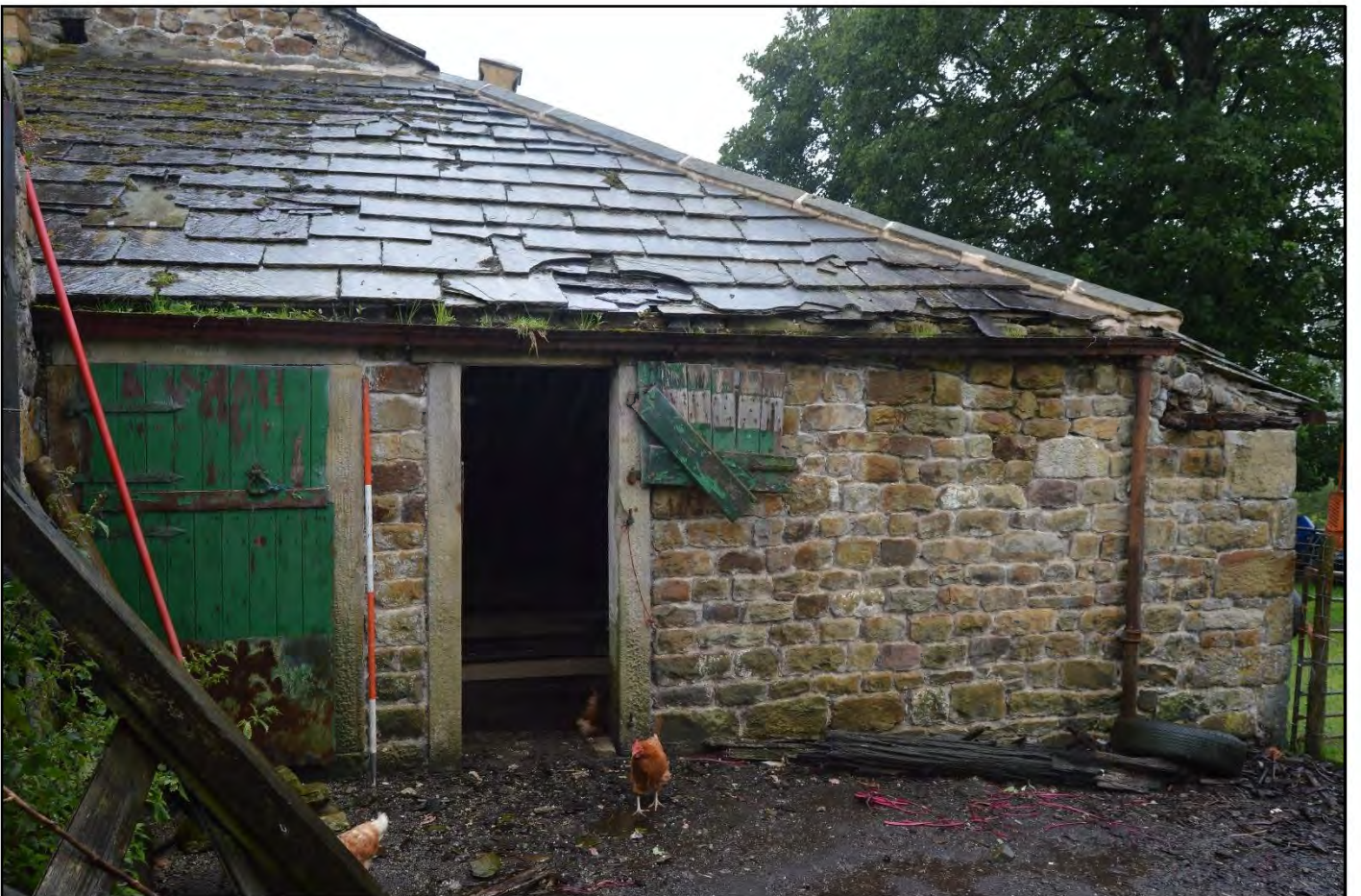
PL18: View of the north east elevation of the shippon to the north west side of the barn.
