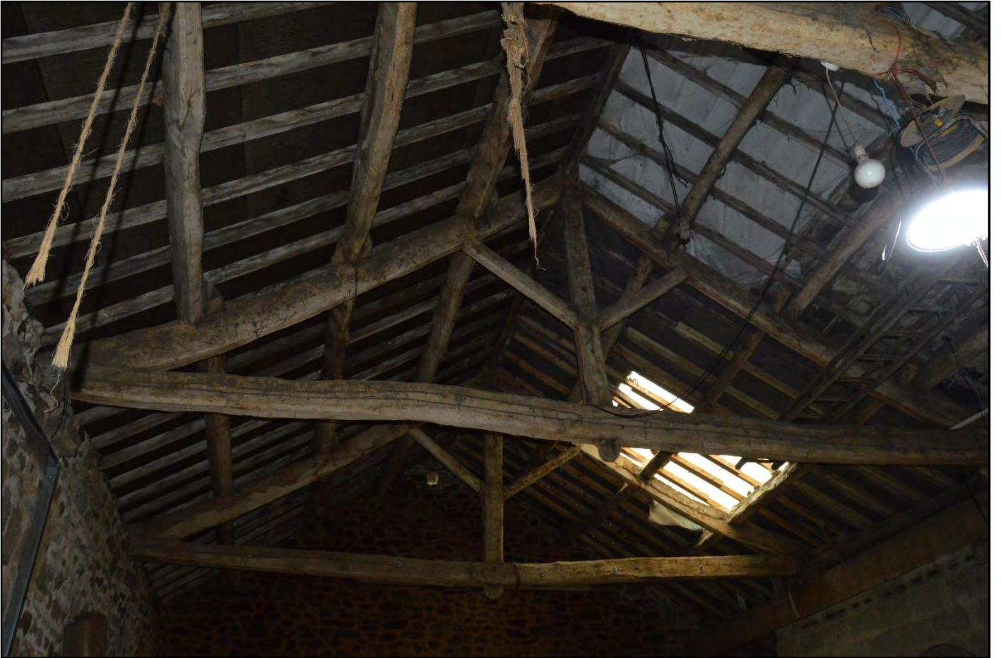
PL38: View of the timber king post roof trusses and associated roof structure preset over the south end of the barn core.
