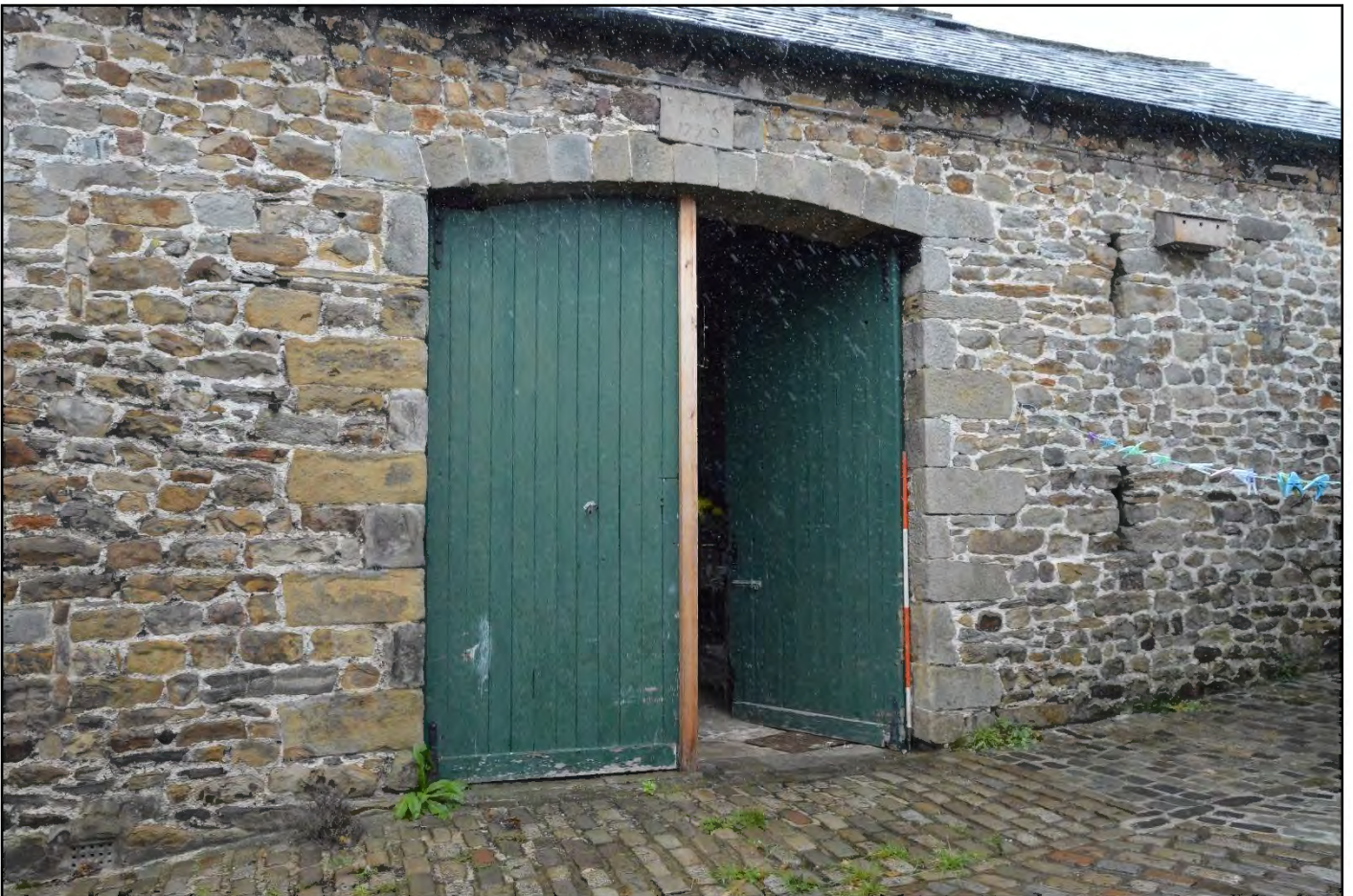
PL02: View of the cart entry doors to the south east elevation of the barn.
