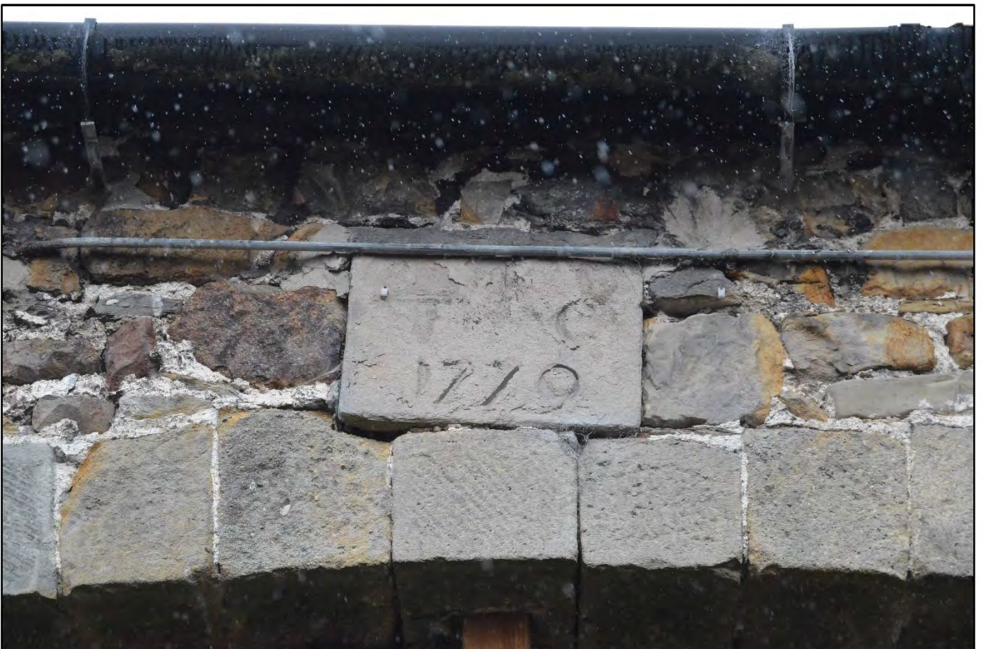
PL04: View of the inscribed datestone over the head of the cart entry doors to the south east elevation of the barn.
