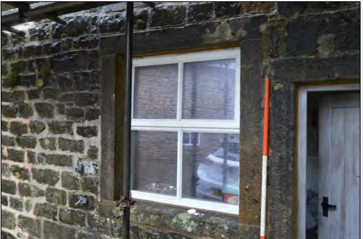
PL57: View of the window to the south west side of the wash house [GF-11].
