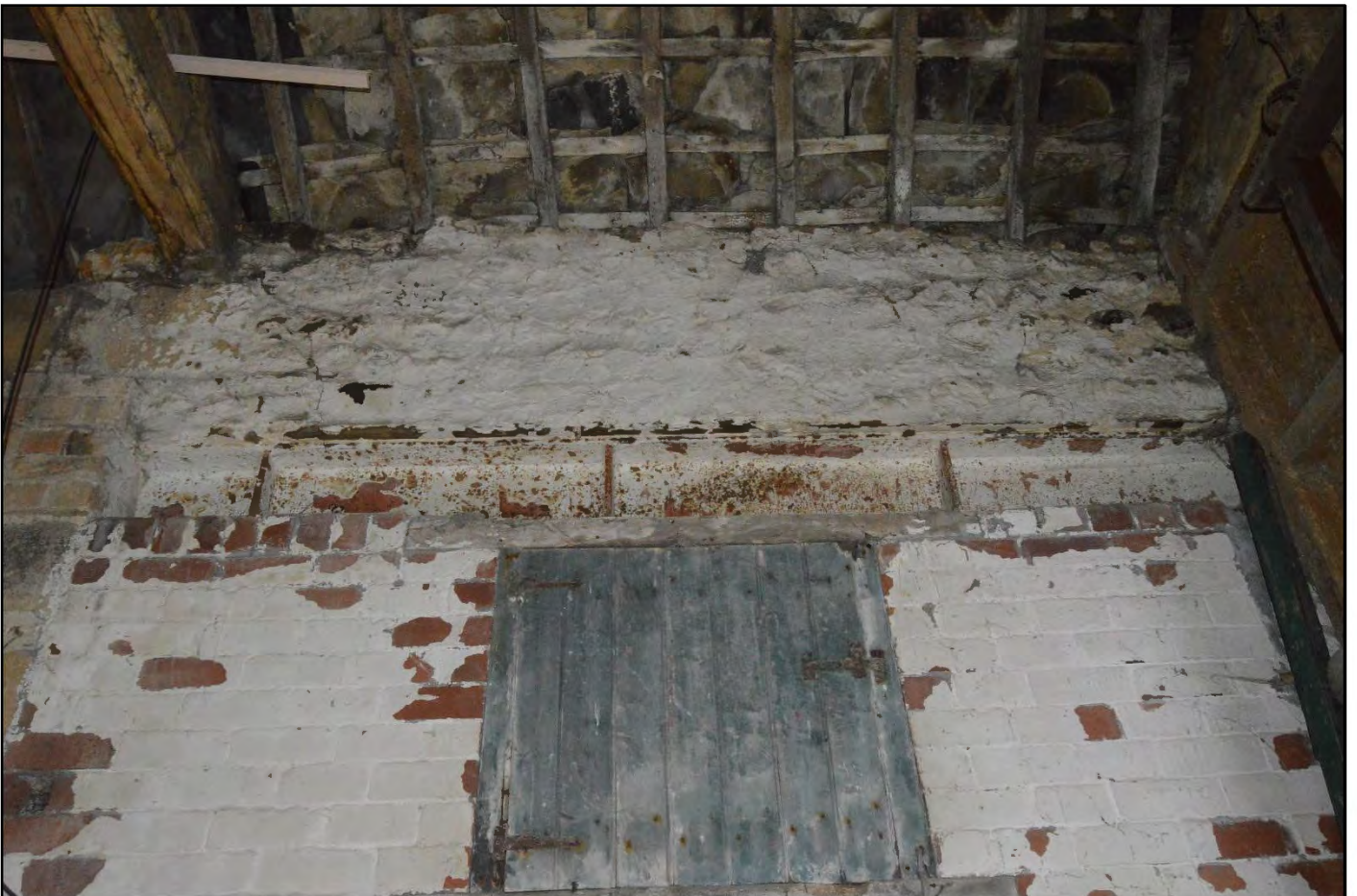
PL37: View of steel beam located above the possible forking hole to the north west side of the barn core.
