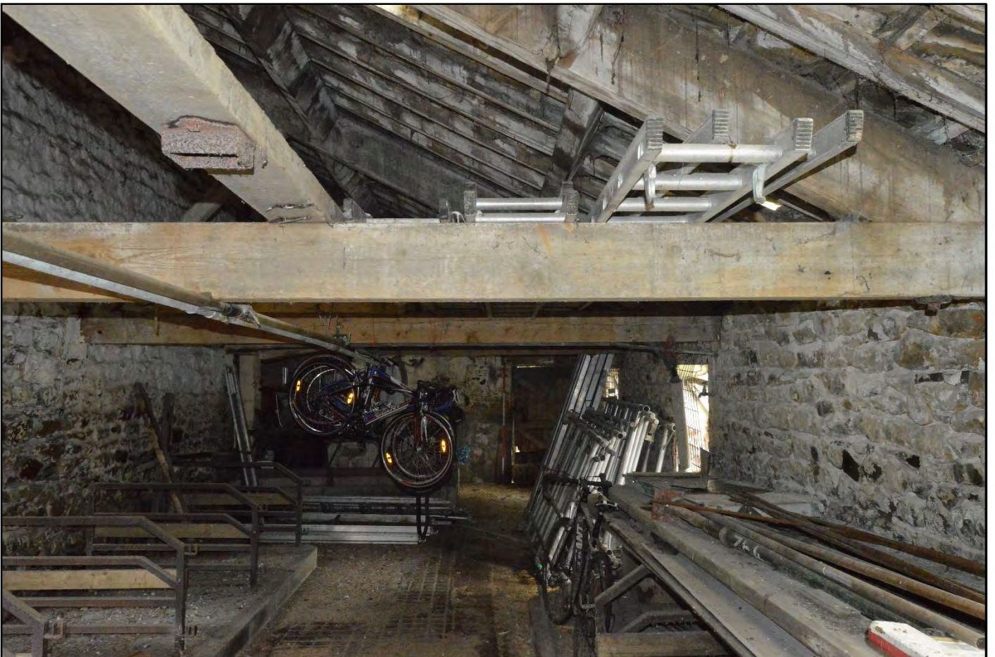
PL41: View south west along the shippon to north west side of the barn [GF-03].
