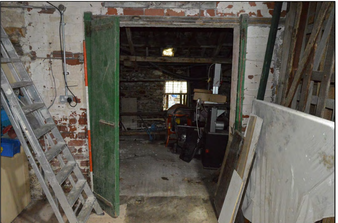
PL35: View of the internal doorway located to the north west side of the barn core, opposite the south east cart entry [GF-04].
