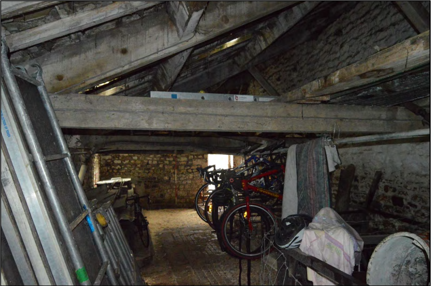
PL40: View north east along the shippon to north west side of the barn [GF-03].
