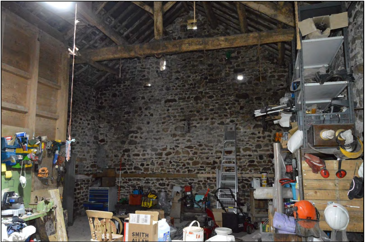
PL30: View north within the barn towards the former hay mew [GF-05].
