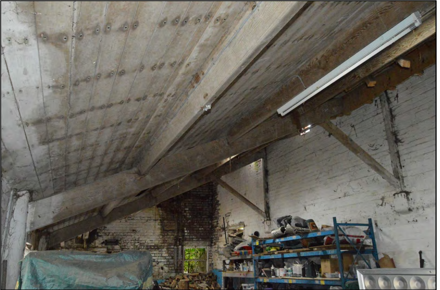
PL74: View of the timber roof structure over the former milking parlour [GF-08].
