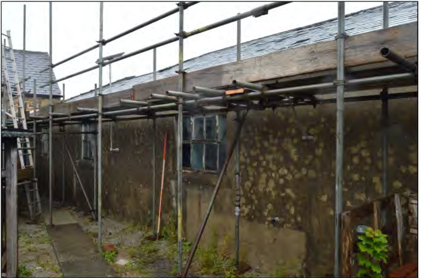
PL66: View of the south elevation of the former ming parlour [GF-08] and wood store [GF-09] from the east.
