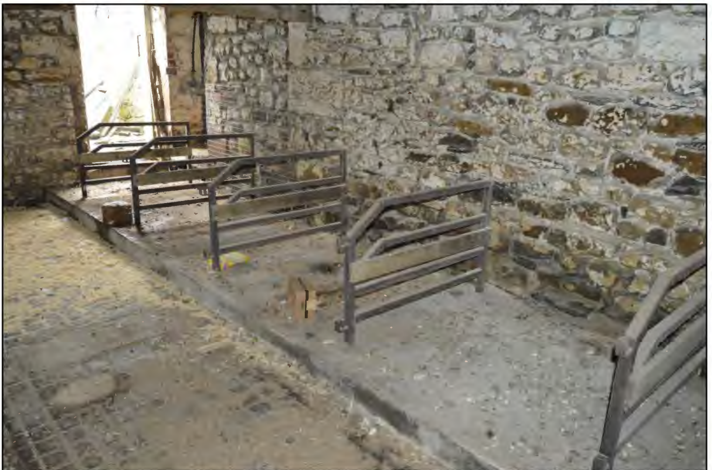
PL46: View of the stalls to the east side of the shippon [GF-03].
