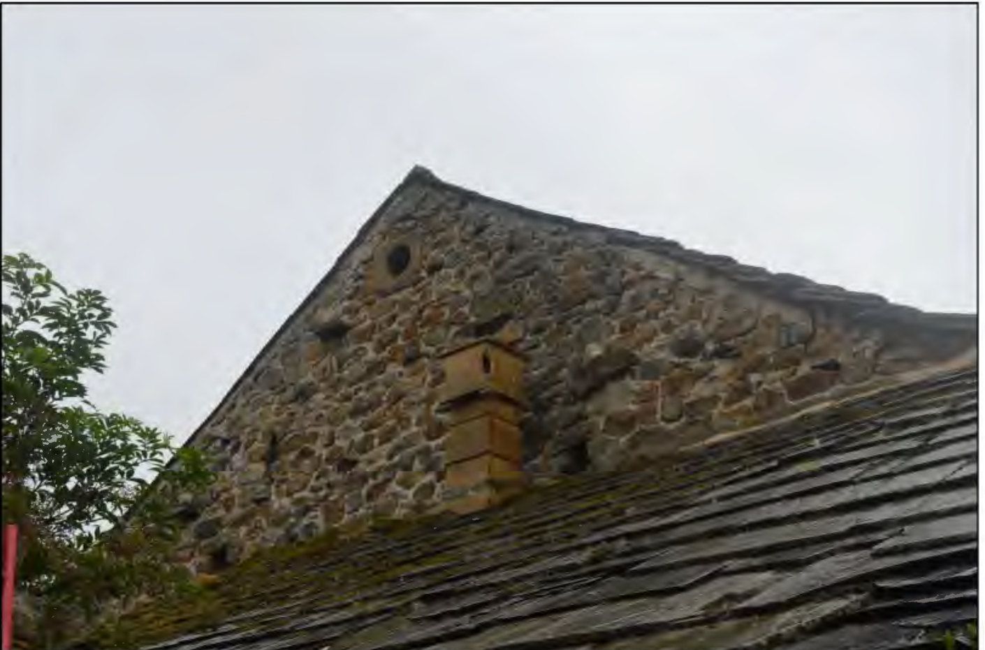
PL21: View of the exposed north east gable end of the barn from the north west.
