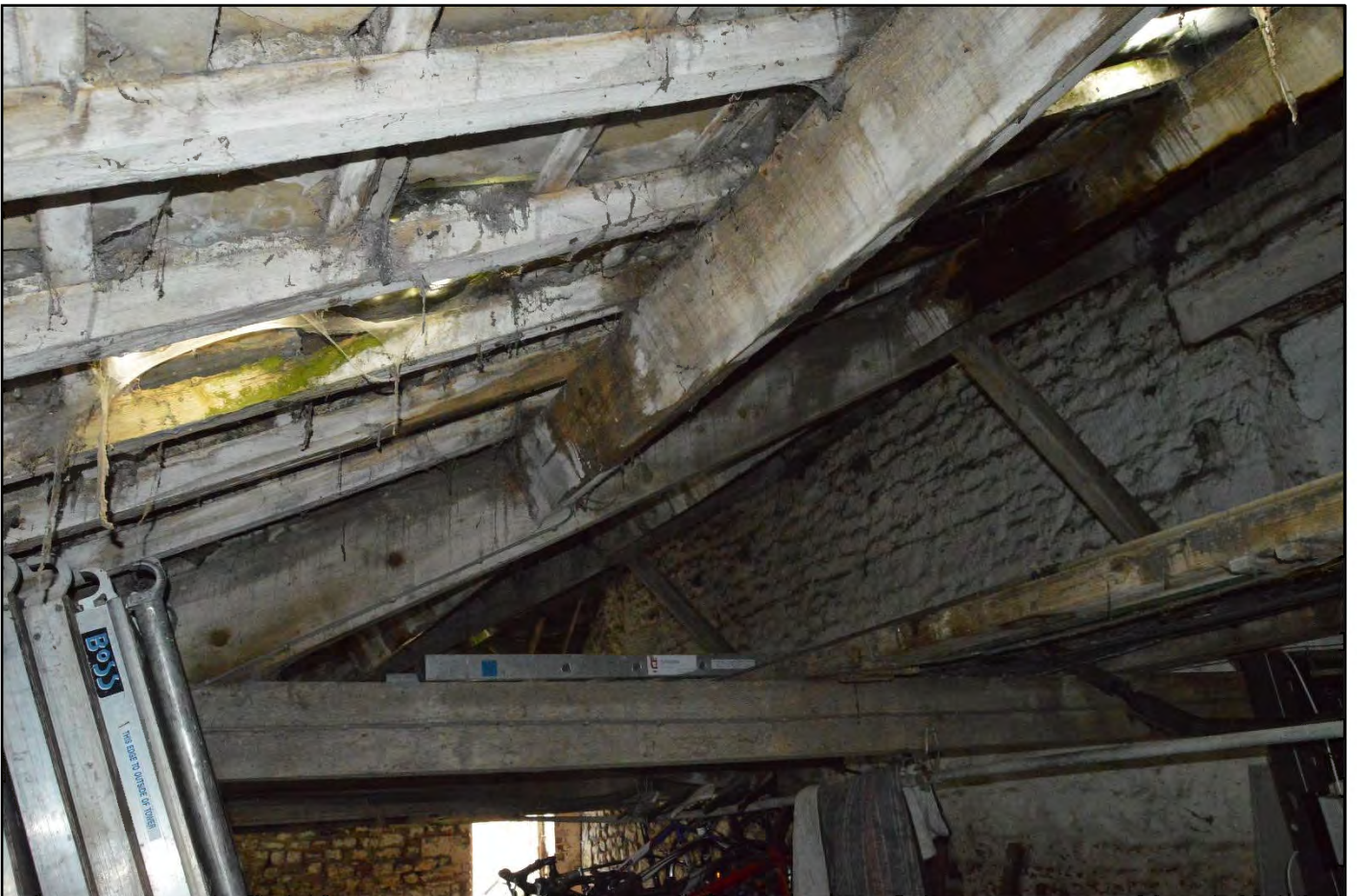
PL48: View of the lean-to roof trusses and associated roof structure to the shippon [GF-03].
