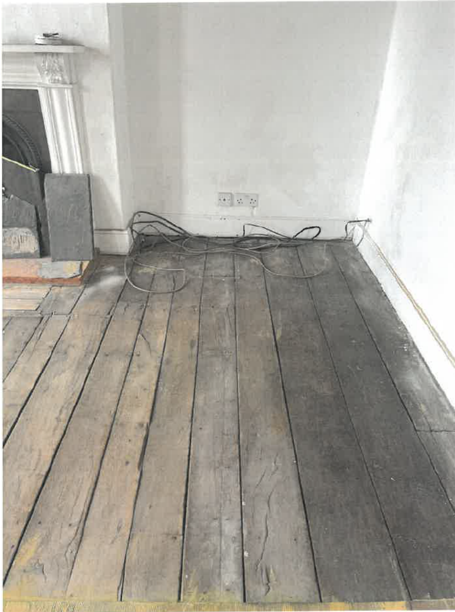
Photograph 5 – General Room View
