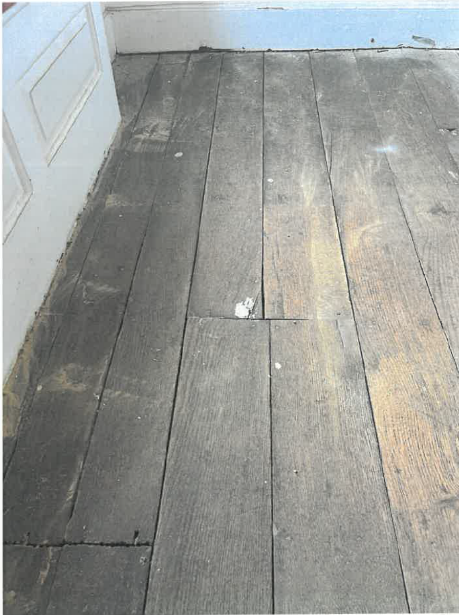
Photograph 7 – Existing Floor Prior to Exposure
