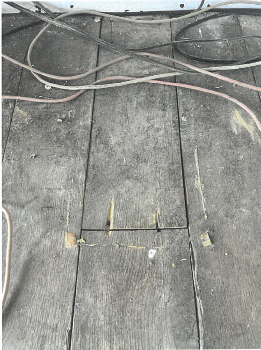
Photograph 3 – Historic Repairs and Alterations
