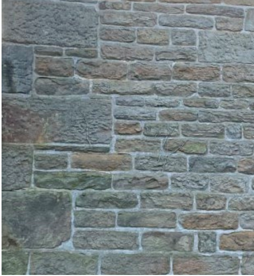
walls - natural stone
