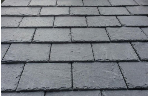
roof - natural slate
