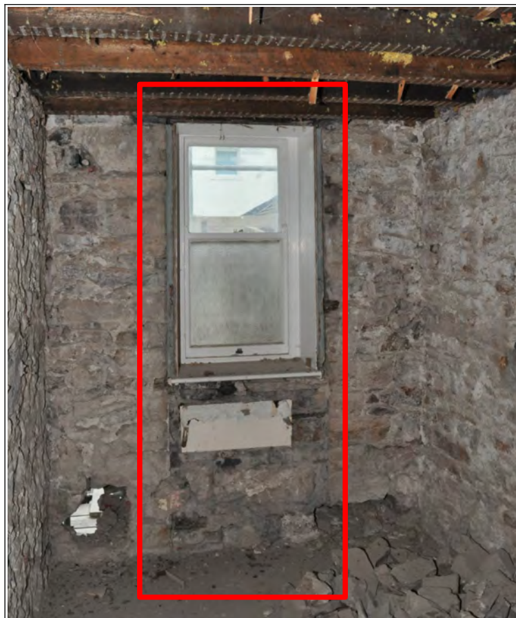
Photo 2: Existing window at first floor level; note infill below
