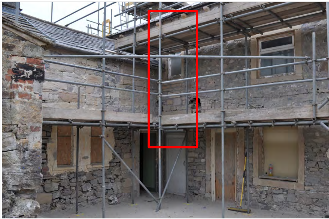
Photo 1: Rear elevation, showing stair window
