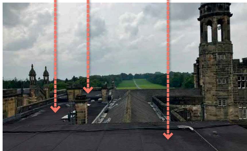
Reverse view from rear quadrangle roof
