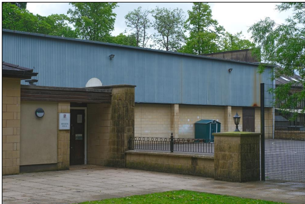
Image showing external view of Building 3 (red arrow) with mature trees and vegetation behind and in close proximity
