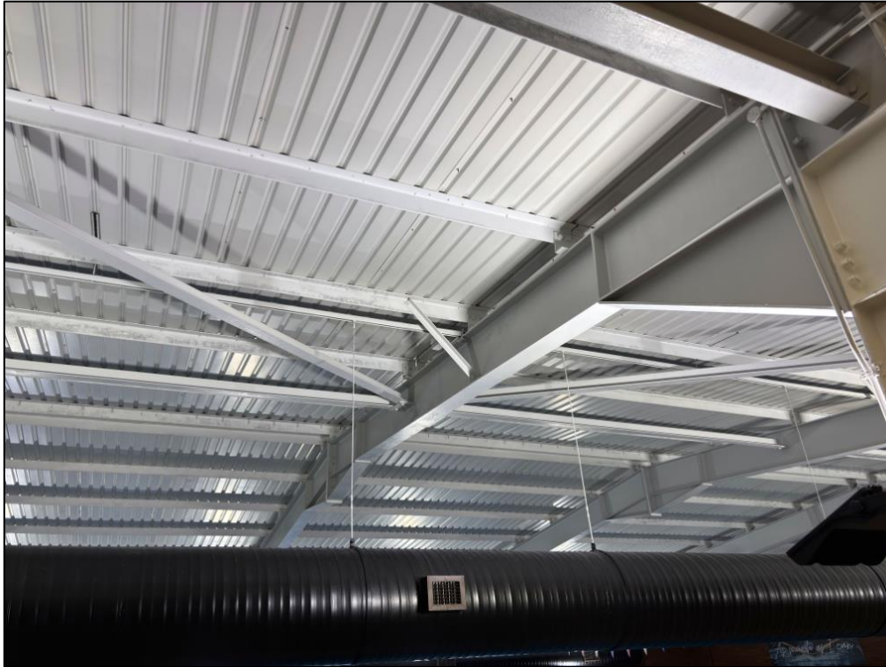
Image showing (internal) roof underside of Building 2
