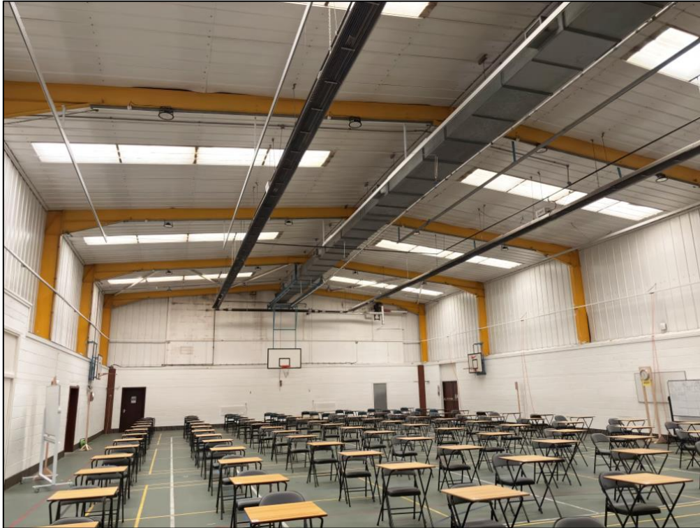
Image showing (internal) roof underside of Building 3
