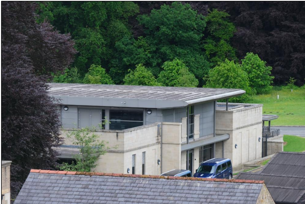
Image showing (external) roof covering of Building 1
