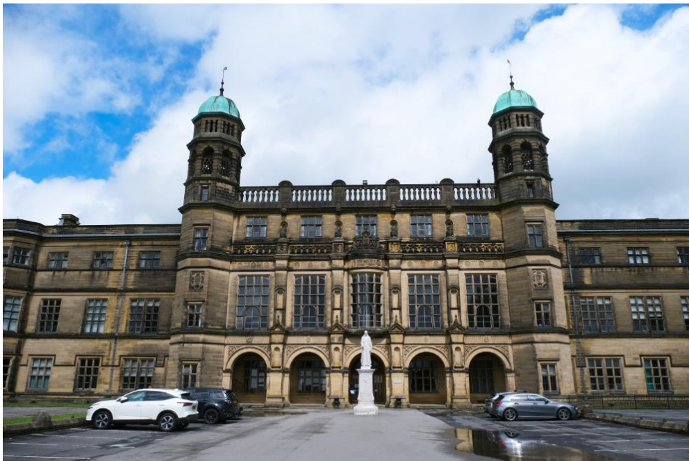
Ground level image of Building 4 showing Towers, known nest site for kestrels
