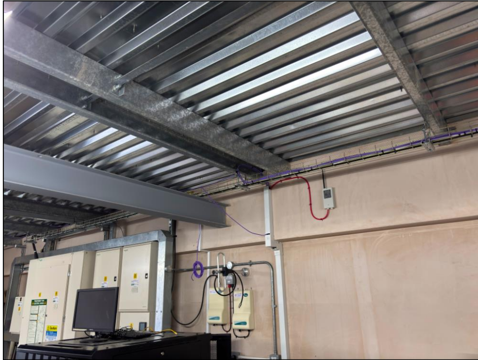
Image showing (internal) roof underside of Building 1
