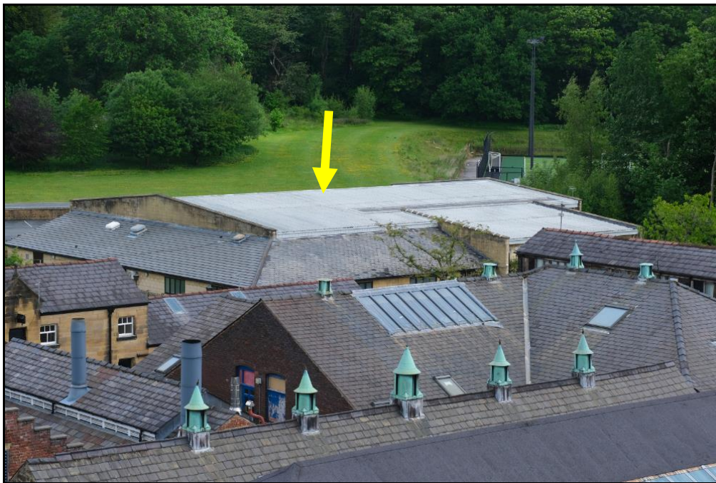
Image 2 – View of Building 2, The Main Sports Centre comprises a shallow pitched metal sheet roof with stone parapet gables and steel roof supports, May 2025
