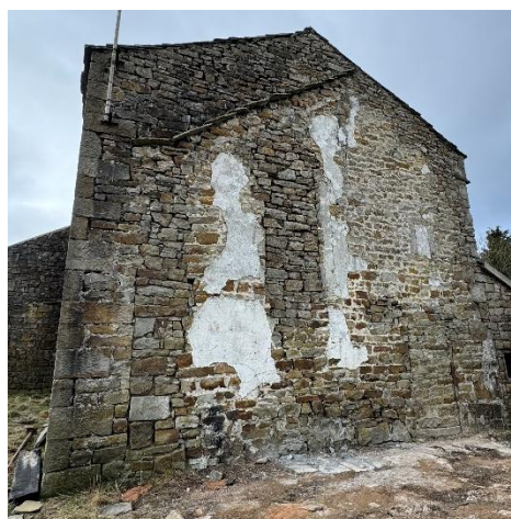
Figure 2 Removed side extension
