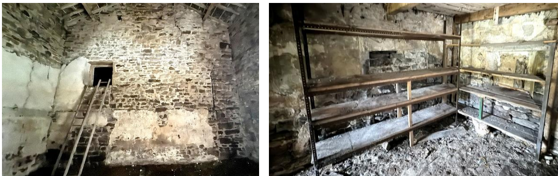
Figure 5 Light shining through roof in areas
