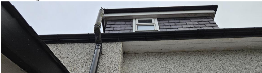
The overhang to the eaves has timber fascia's with boarded soffits.
