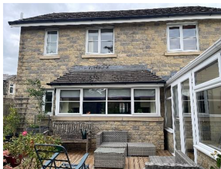
Figure 2: kitchen windows / mono-pitch roof
