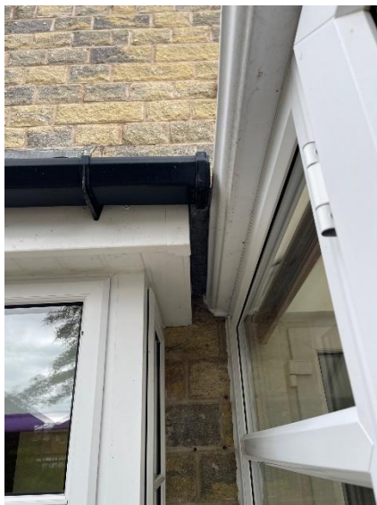
Figure 5: kitchen window / conservatory detail
