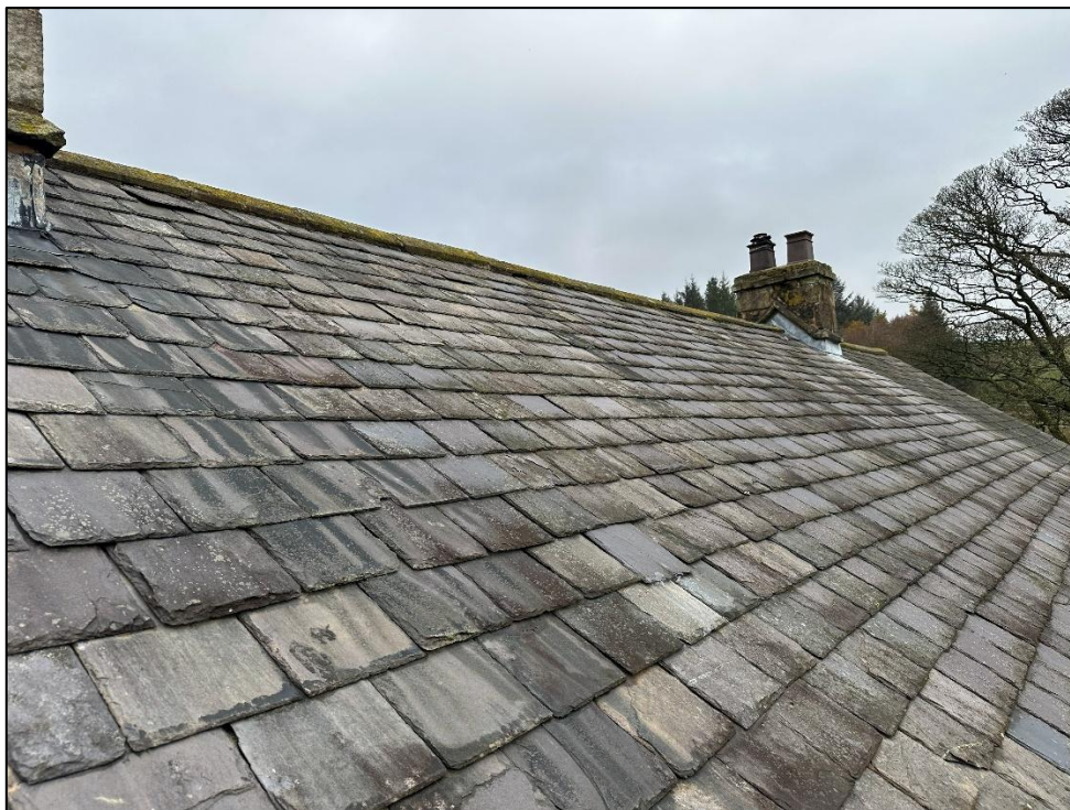
Plate 3: The pitched main roof was in good condition.
