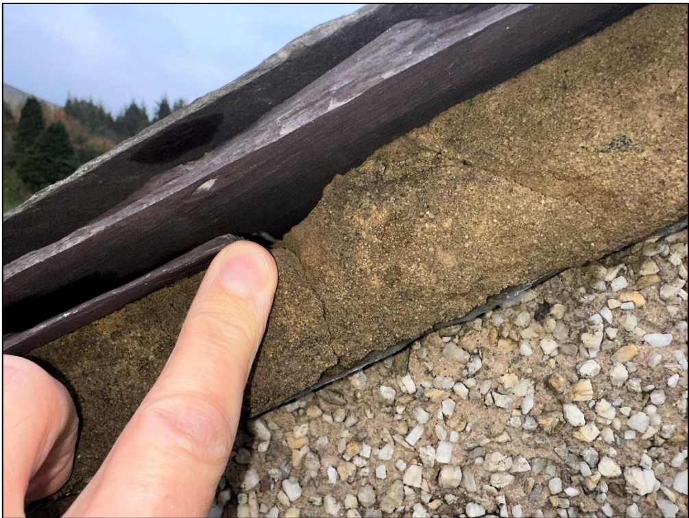
Plate 9: There were some gaps in the verge which, were too small and did not have roosting potential.
