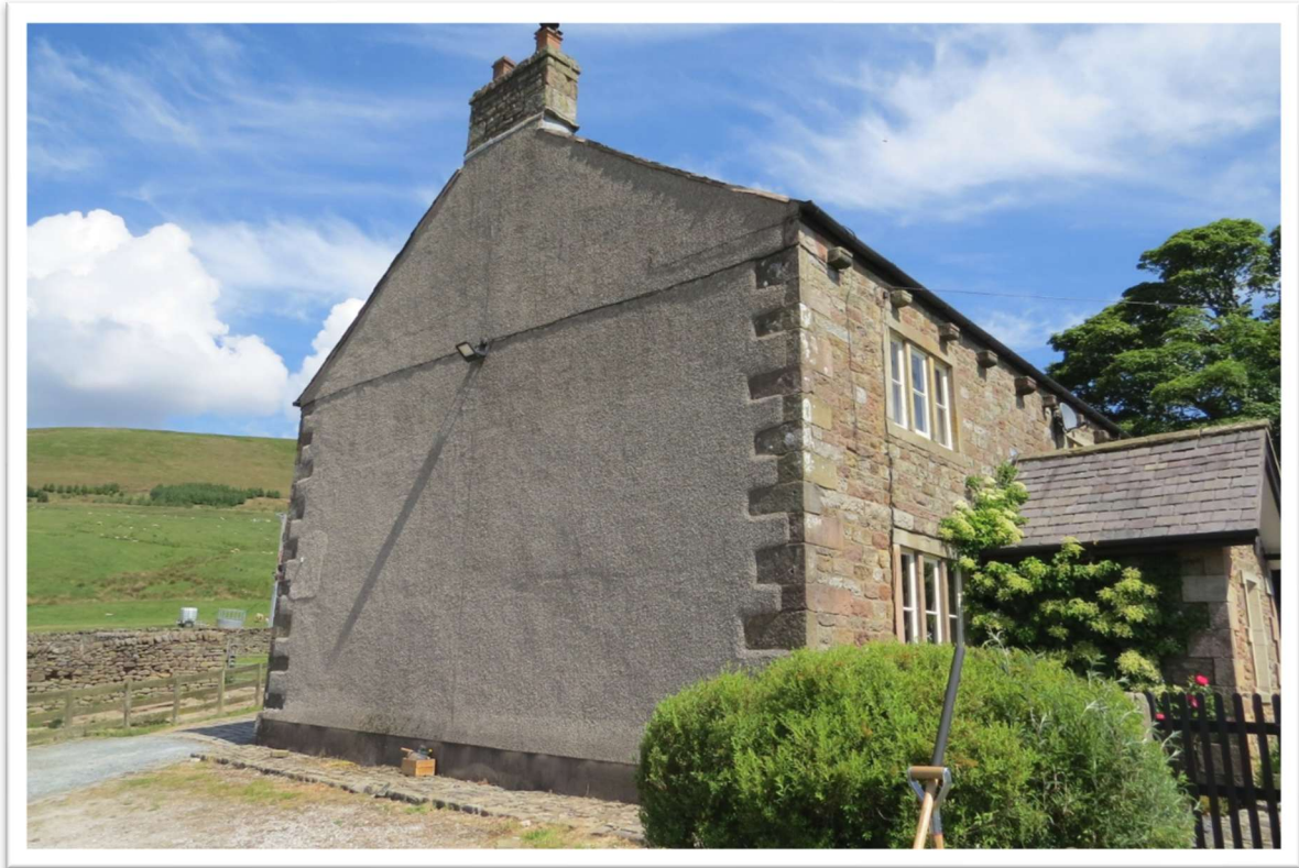
1. Cement render to gable wall
