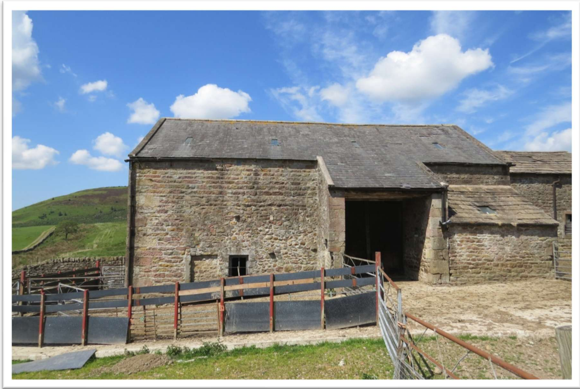
3. Historic barn opposite farmhouse with water tabling to verge
