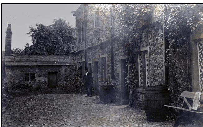
Fig 06: Late 19 th century photograph showing Abbeycroft.
