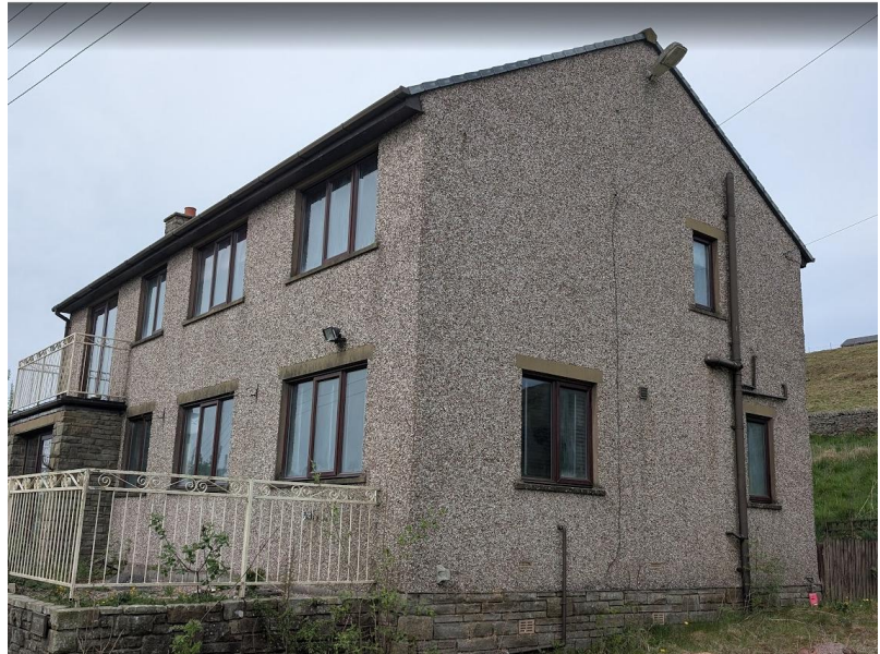
Photo 1. Frontage and north-east gable.
