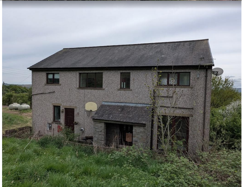
Photo 2. Rear (north-west) aspect.
