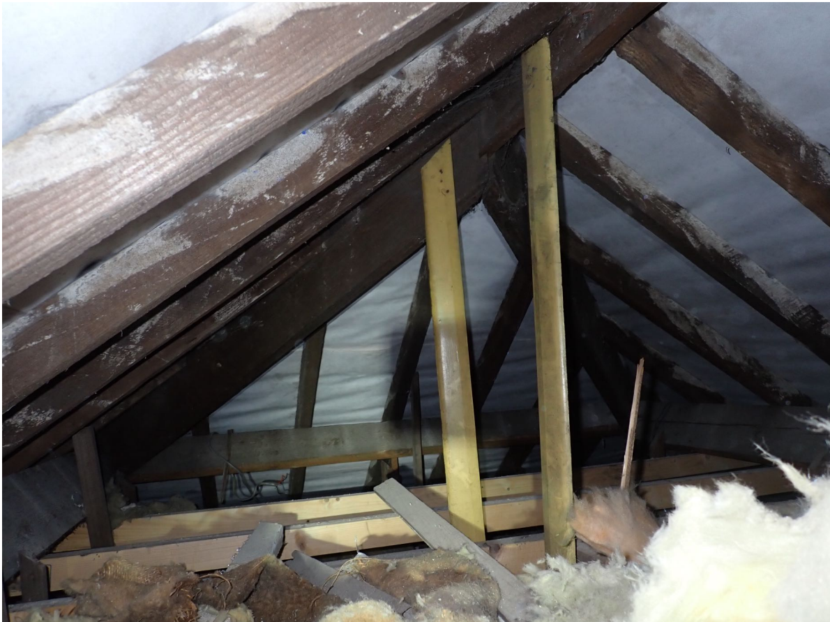
3.2a – The roof void.
