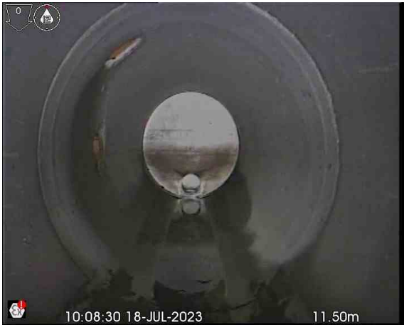
S10X_26fa98fc-5ad2-4dcf-b9d7-36a9c5c48fa0_20230719_083612_351.jpg, 00:00:46, 11.50 m Connection other than junction at 10 o'clock, 150mm dia
