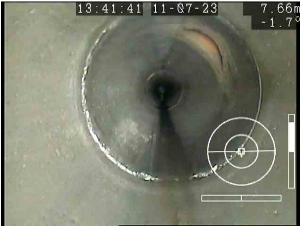
S4X_64431a07-b02a-4f5f-9758-9be73cdd54e8_20230717_123442_232.jpg, 00:00:29, 7.66 m Connection other than junction at 01 o'clock, 150mm dia
