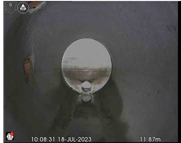
S10X_42a1f004-fcdd-4655-b05e-65b8c754aea6_20230719_083623_583.jpg, 00:00:48, 11.87 m Connection other than junction at 09 o'clock, 150mm dia
