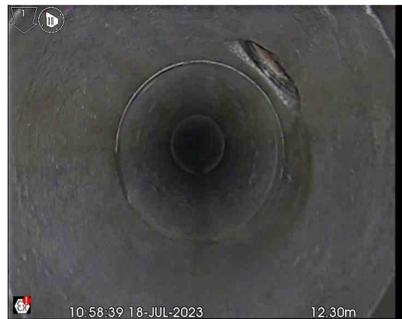
S5X_f910e798-03df-476f-bd0b-94fccaa5d9d2_20230719_083915_260.jpg, 00:00:50, 12.30 m Connection other than junction at 01 o'clock, 150mm dia
