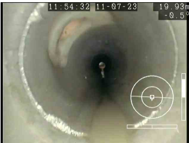
S2X_of3c6b7a-adf1-44ce-ac15-979ad2b0b05e_20230717_12 2945_776.jpg, 00:01:02, 19.93 m Connection other than junction at 11 o'clock, 150mm dia
