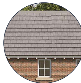
Exposed rafter feet
