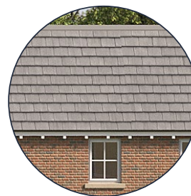
Exposed rafter feet
