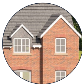
Projecting gable and dormer
