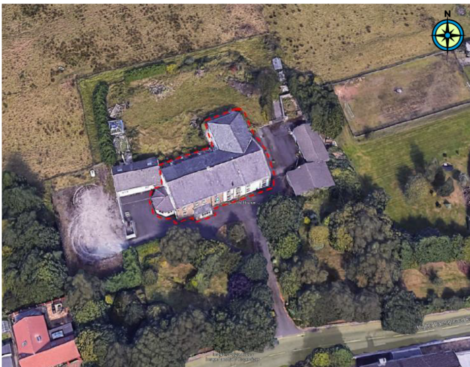
Figure 1.1: Aerial image of building at Longworth House, Blackburn.
