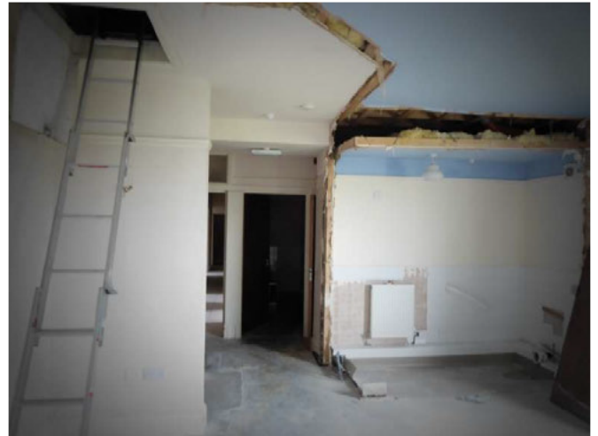
Typical internal first floor areas.
