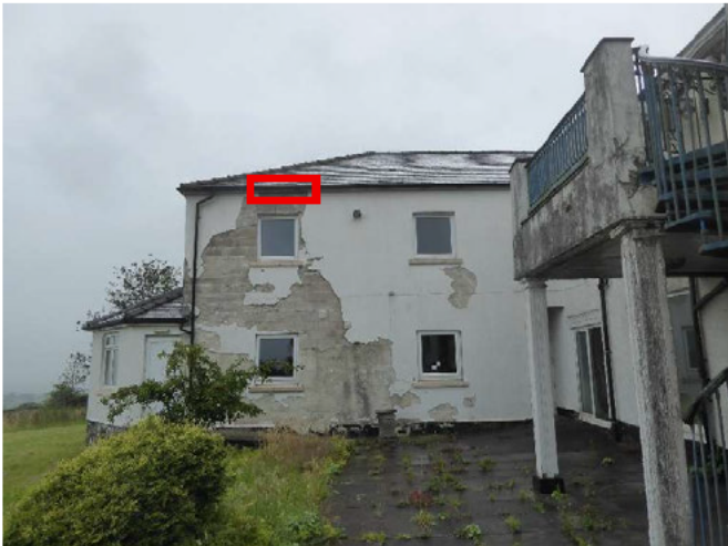
Wing of property extending north with bat roost potential (see below);
