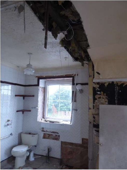
Typical internal first floor areas.
