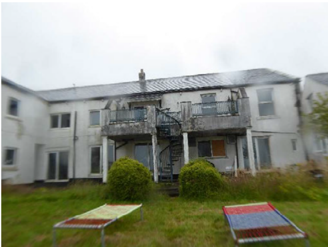
Rear NW elevation, general view.
