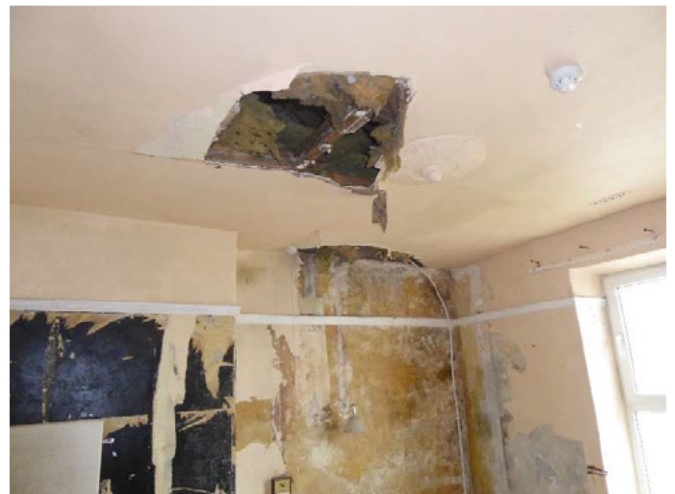
Typical internal first floor areas.
