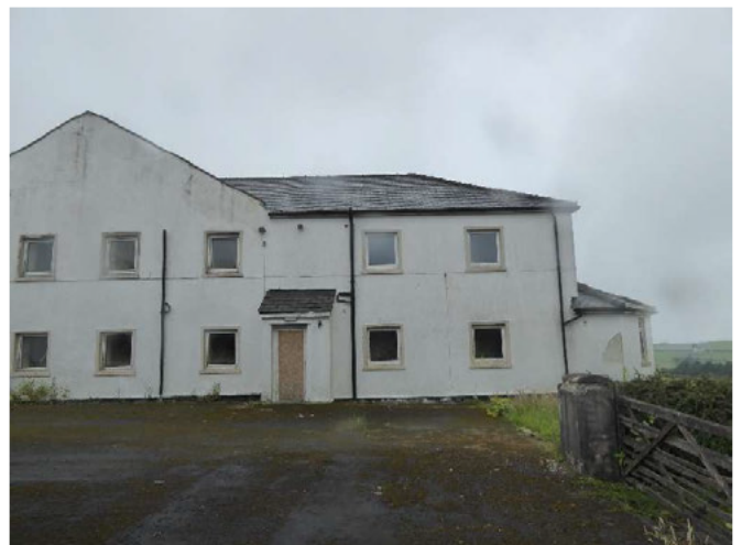
Side NE elevation general view, no potential bat roost features.
