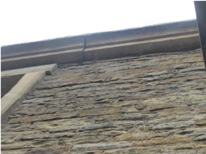
SE front elevation stone fascia fits tight to wall plate, no gaps.
