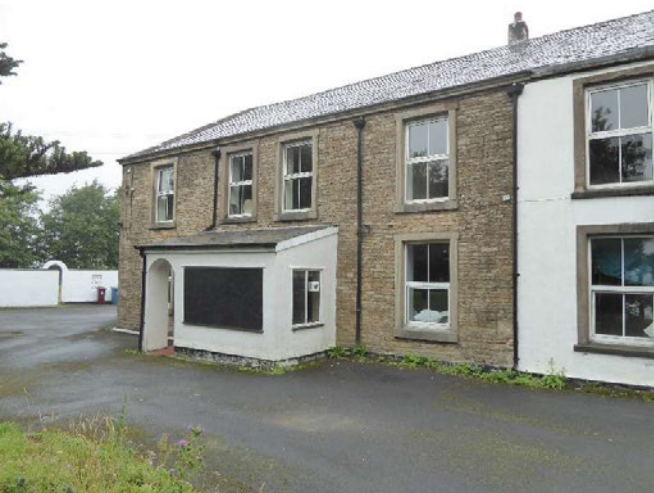
Front SE elevation (eastern end).
