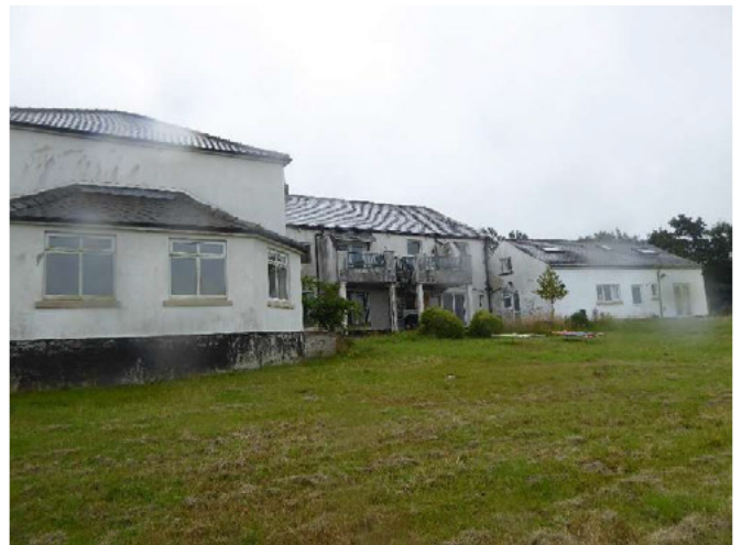
Rear NW elevation general view.
