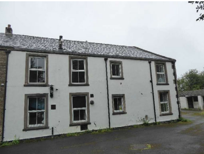
Front SE elevation (eastern end).
