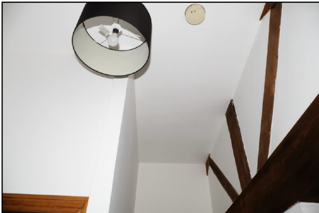
Image showing vaulted ceiling in first floor stairwell.
