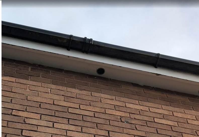
Photo 4. Example of soffits well sealed to the walls.
