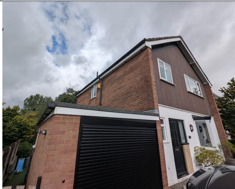
Photo 2. Front and side elevation (area of extension).
