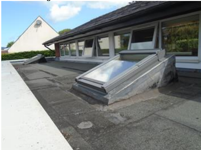
Flat roof with parapet wall
