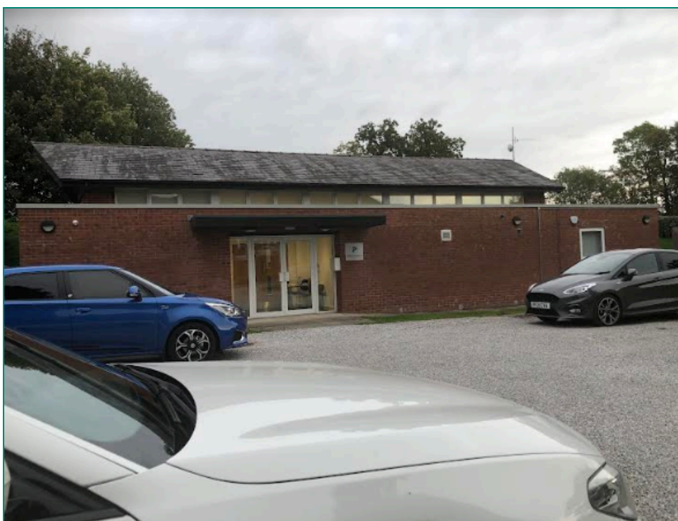
Figure 1 - Photograph of existing building (front)
