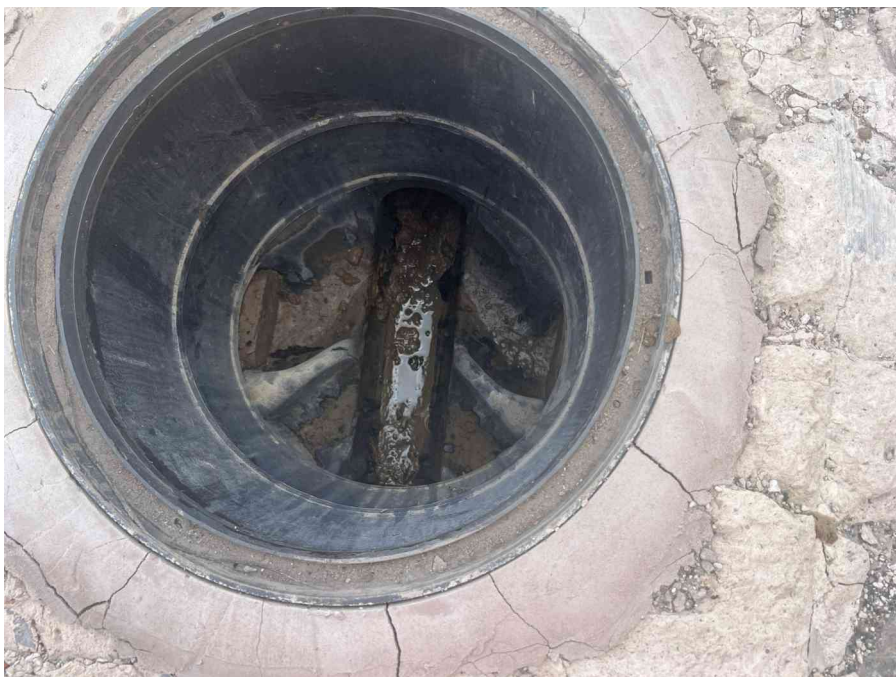
MH09X_D_14082025_1220_049.jpg, 00:00:00, 0.00 m Start node, inspection chamber, reference: MH09, IC LOCATED ADJACENT TO BAY DOORS
