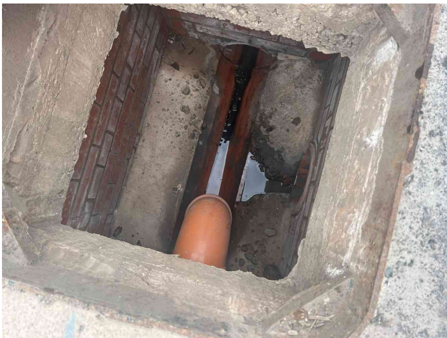
MH07X_U_14082025_1229_054.jpg, 00:00:00, 0.00 m Start node, manhole, reference: MH08, MANHOLE LOCATED ADJACENT TO LOADING BAY
