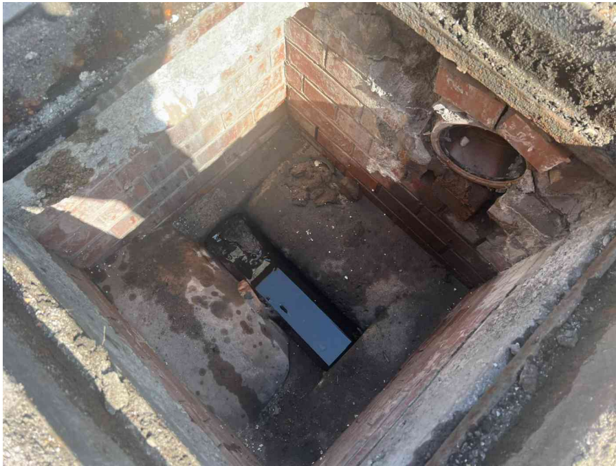
MH01X_D_13082025_0951_005.jpg, 00:00:30, 2.99 m Finish node, manhole, reference: MH02, MANHOLE LOCATED ADJACENT TO STAIRCASE
