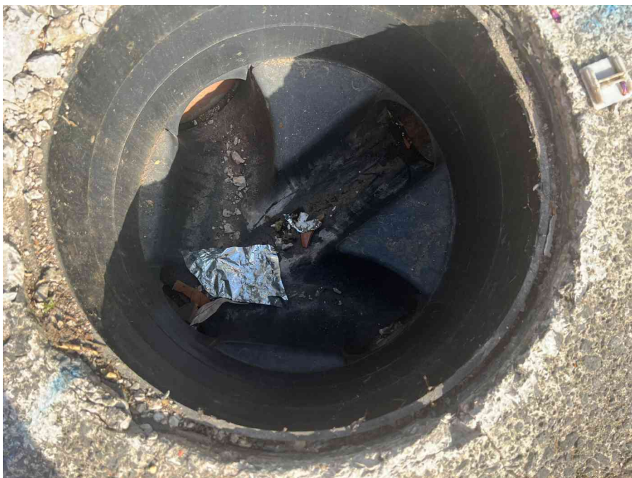
MH01AX_U_13082025_0954_007.jpg, 00:00:00, 0.00 m Start node, inspection chamber, reference: MH01, IC LOCATED ADJACENT TO STAIR CASE
