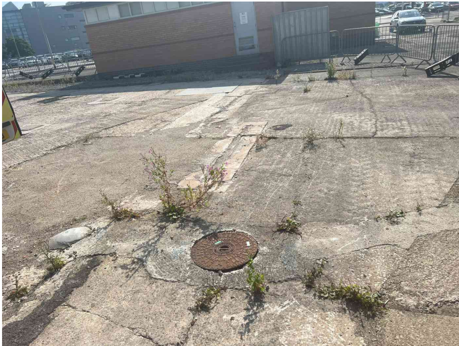
MH01AX_U_13082025_0954_006.jpg, 00:00:00, 0.00 m Start node, inspection chamber, reference: MH01, IC LOCATED ADJACENT TO STAIR CASE
