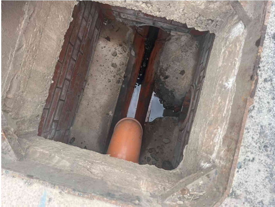
MH09X_D_14082025_1220_052.jpg, 00:00:27, 2.48 m Finish node, manhole, reference: MH08
