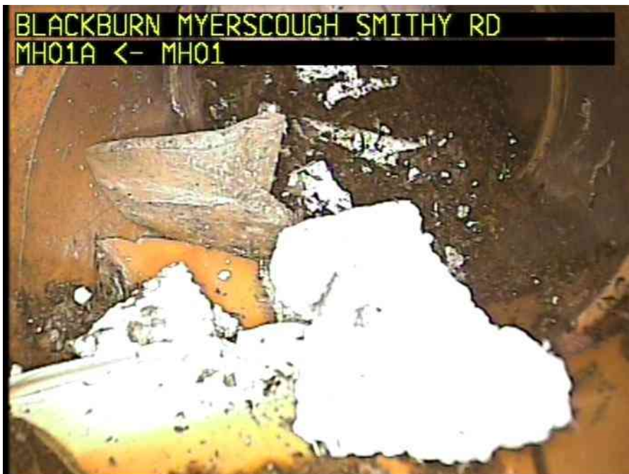
MH01AX_U_13082025_0954_009.jpg, 00:00:24, 1.02 m Line deviates up
