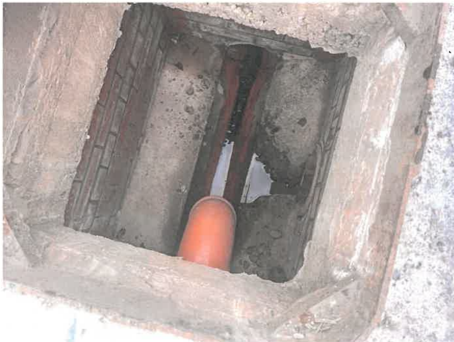
MH08X_D_14082025_1244_073.jpg, 00:00:00, 0.00 m Start node, manhole, reference: MH08, MANHOLE LOCATED ADJACENT TO LOADING BAY DOOR.
