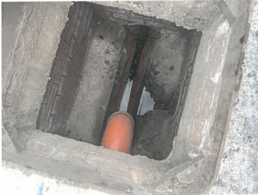
MH09X_D_14082025_1220_052.jpg, 00:00:27, 2.48 m Finish node, manhole, reference: MH08
