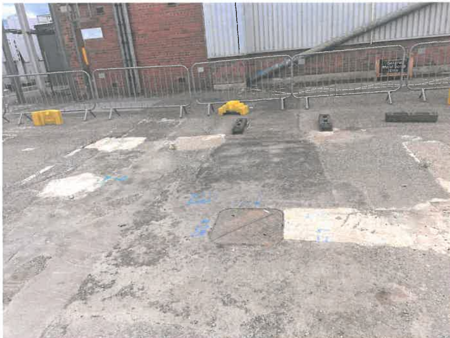
MH09X_D_14082025_1220_051.jpg, 00:00:27, 2.48 m Finish node, manhole, reference: MH08
