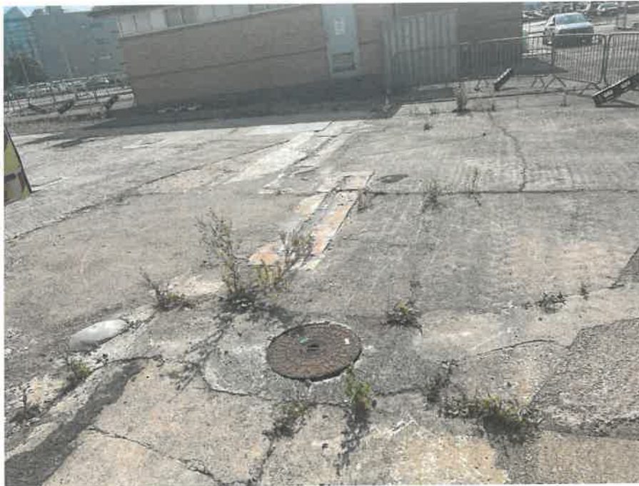
MH01AX_U_13082025_0954_006.jpg, 00:00:00, 0.00 m Start node, inspection chamber, reference: MH01, IC LOCATED ADJACENT TO STAIR CASE
