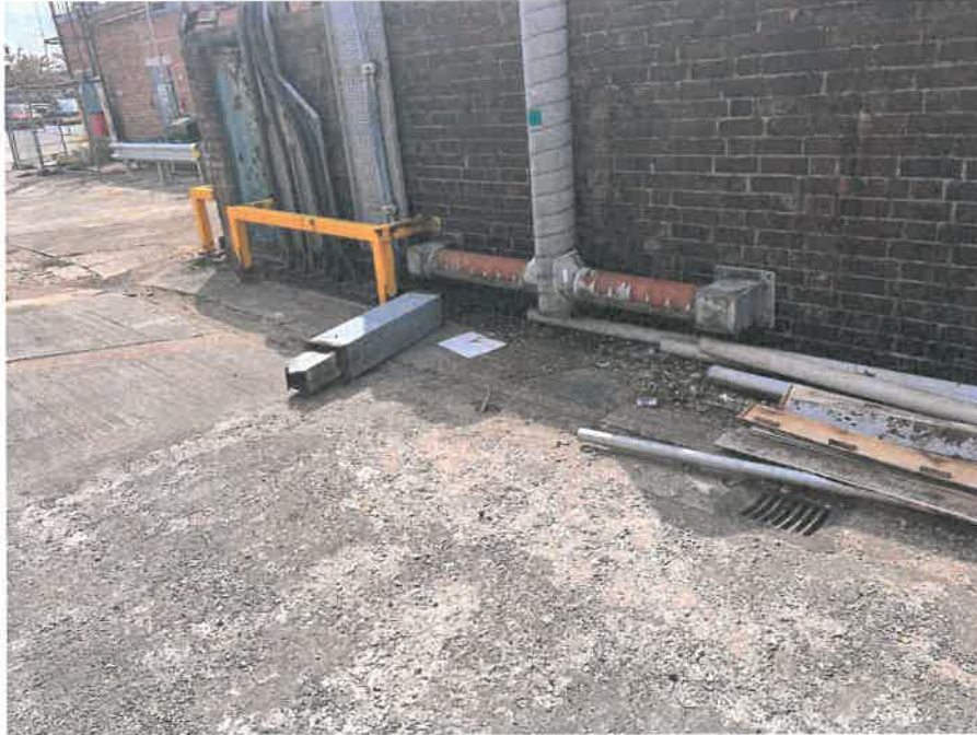
MH04AX_U_13082025_1217_039.jpg, 00:00:00, 0.00 m Start node, manhole, reference: MH04, MANHOLE LOCATED ADJACENT TO DUCTING
