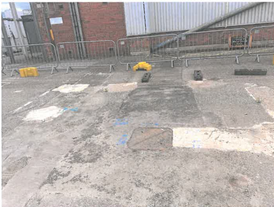
MH08AX_U_14082025_1232_064.jpg, 00:00:00, 0.00 m Start node, manhole, reference: MH08, MANHOLE LOCATED ADJACENT TO LOADING BAY
