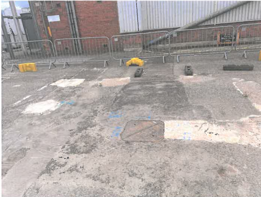
MH08X_D_14082025_1244_072.jpg, 00:00:00, 0.00 m Start node, manhole, reference: MH08, MANHOLE LOCATED ADJACENT TO LOADING BAY DOOR.
