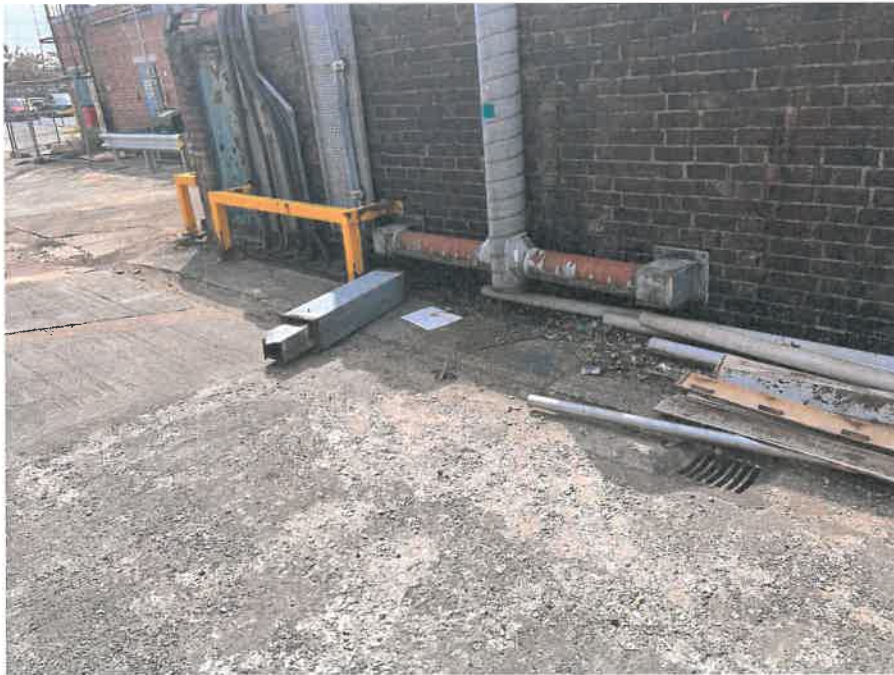
MH04BX_U_13082025_1225_045.jpg, 00:00:00, 0.00 m Start node, manhole, reference: MH04, MANHOLE LOCATED ADJACENT TO DUCTING
