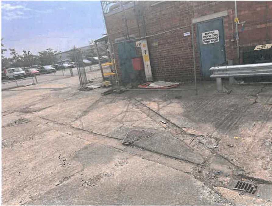
MH04X_D_13082025_1054_031.jpg, 00:01:33, 14.17 m Finish node, manhole, reference: MH05, MANHOLE LOCATED ADJACENT TO FIRE EXIT
