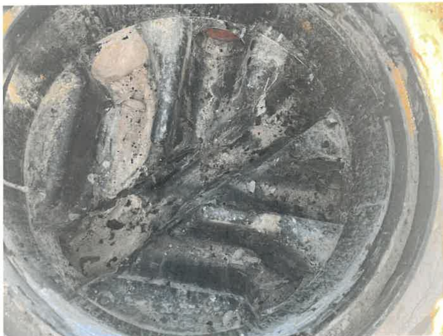
MH06X_D_13082025_1145_034.jpg, 00:00:00, 0.00 m Start node, inspection chamber, reference: MH06, IC LOCATED ADJACENT TO FILTER STORES
