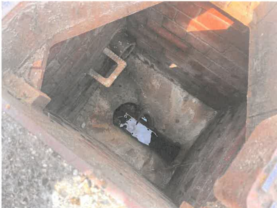
MH04X_D_13082025_1054_032.jpg, 00:01:33, 14.17 m Finish node, manhole, reference: MH05, MANHOLE LOCATED ADJACENT TO FIRE EXIT
