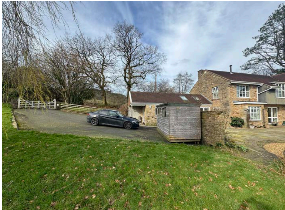
Figure 4. Sloped South Access
