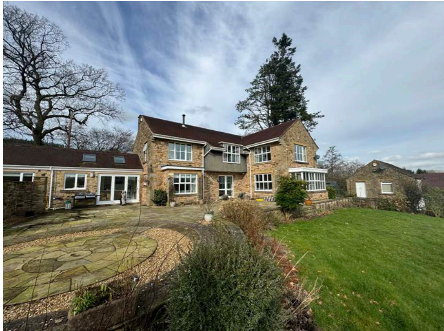
Figure 3. South East elevation
