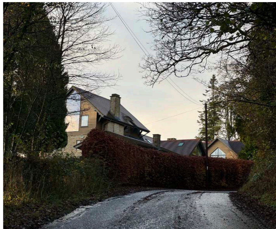
Figures 10,11. Sagar Wood: prominent glazing and non-stone cladding
