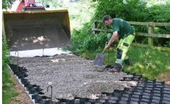
Figure 7: Application of membrane and stone confinement system to allow for a minimal dig approach to installation of roadways and parking areas. This reduces soil damage, reducing effects on site hydrology, and protects tree roots from severance or crushing. It also requires the use of a lot less stone to form a solid base for these structures. Image courtesy of CellWeb™, 2022.
