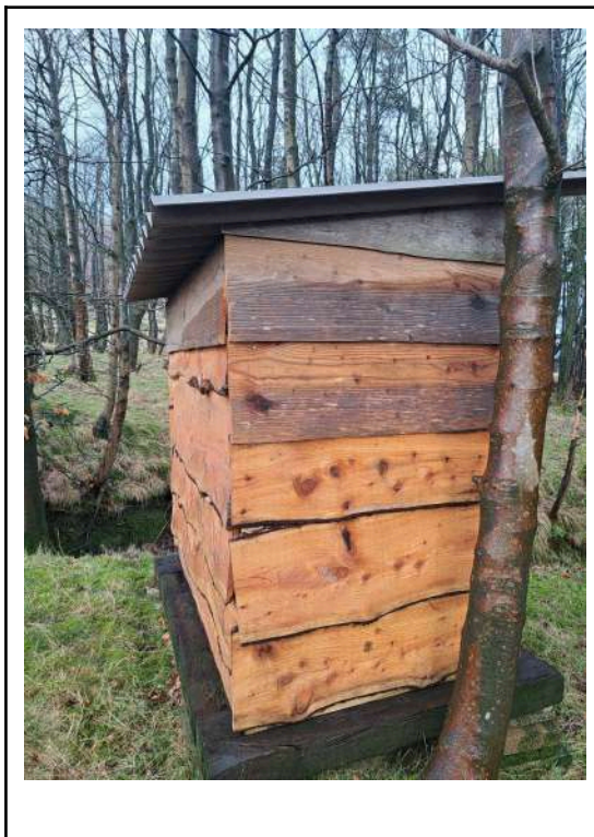
Photograph 1- External of timber out house
