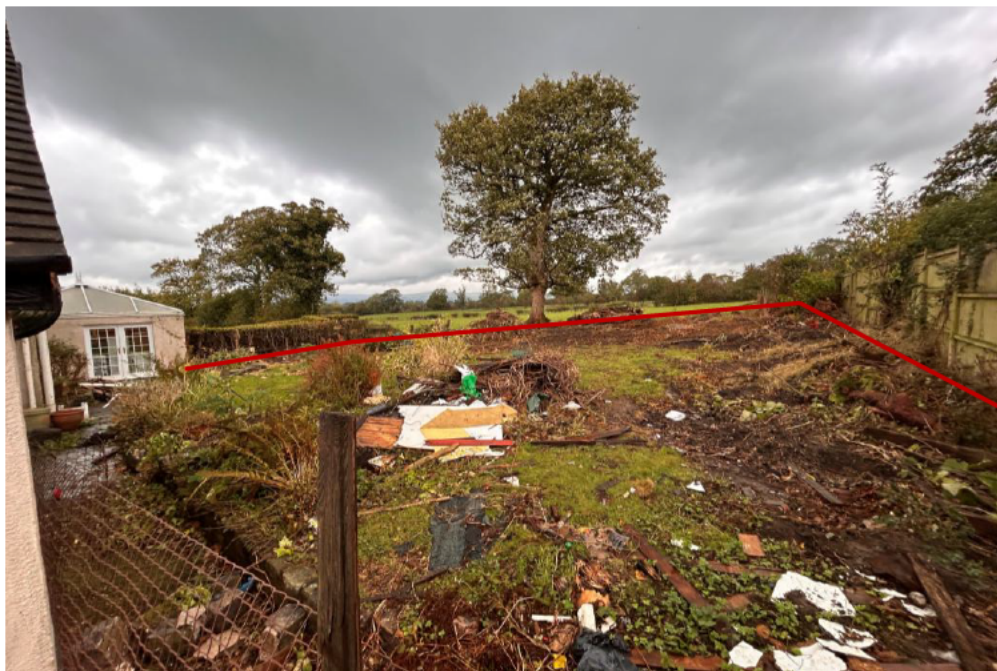
Rear of Site – Site Cleared
