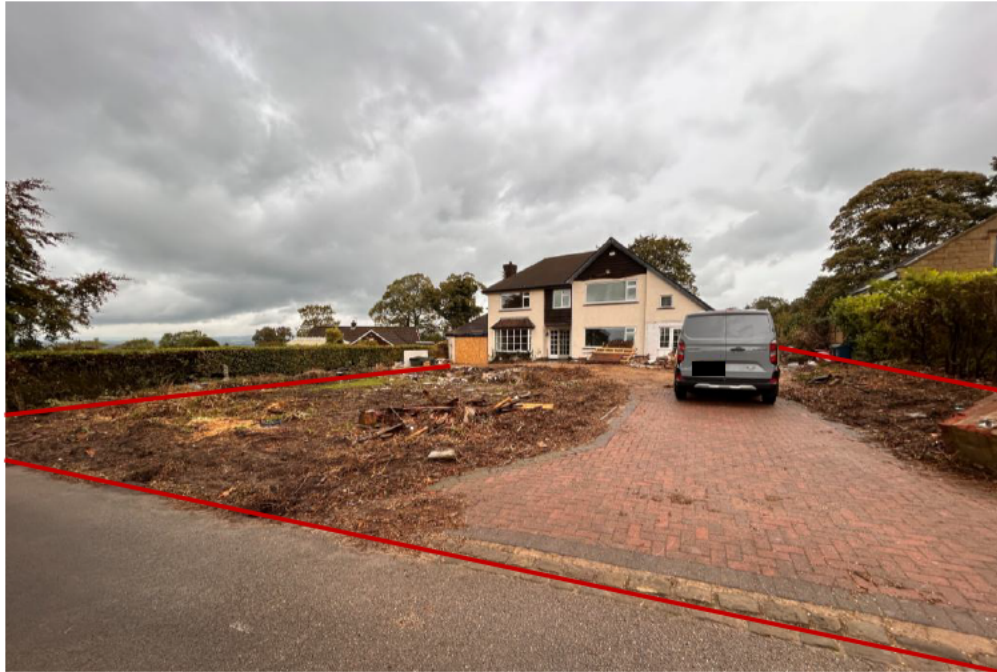
Front of Site – Site Cleared
