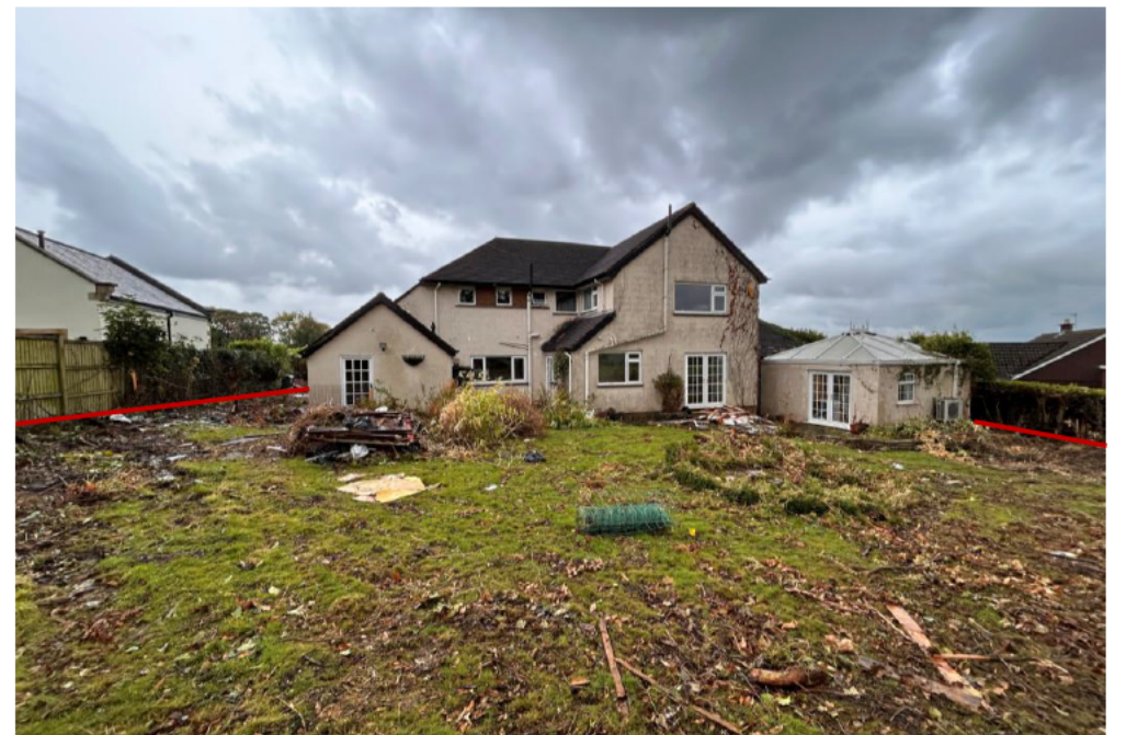
Rear of Site – Site Cleared
