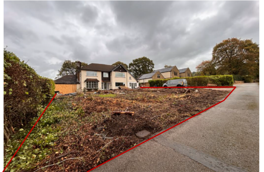
Front of Site – Site Cleared
