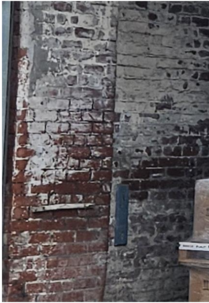
Brick wall internal
