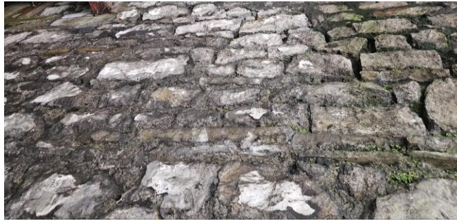
Stone mill wall (retained)
