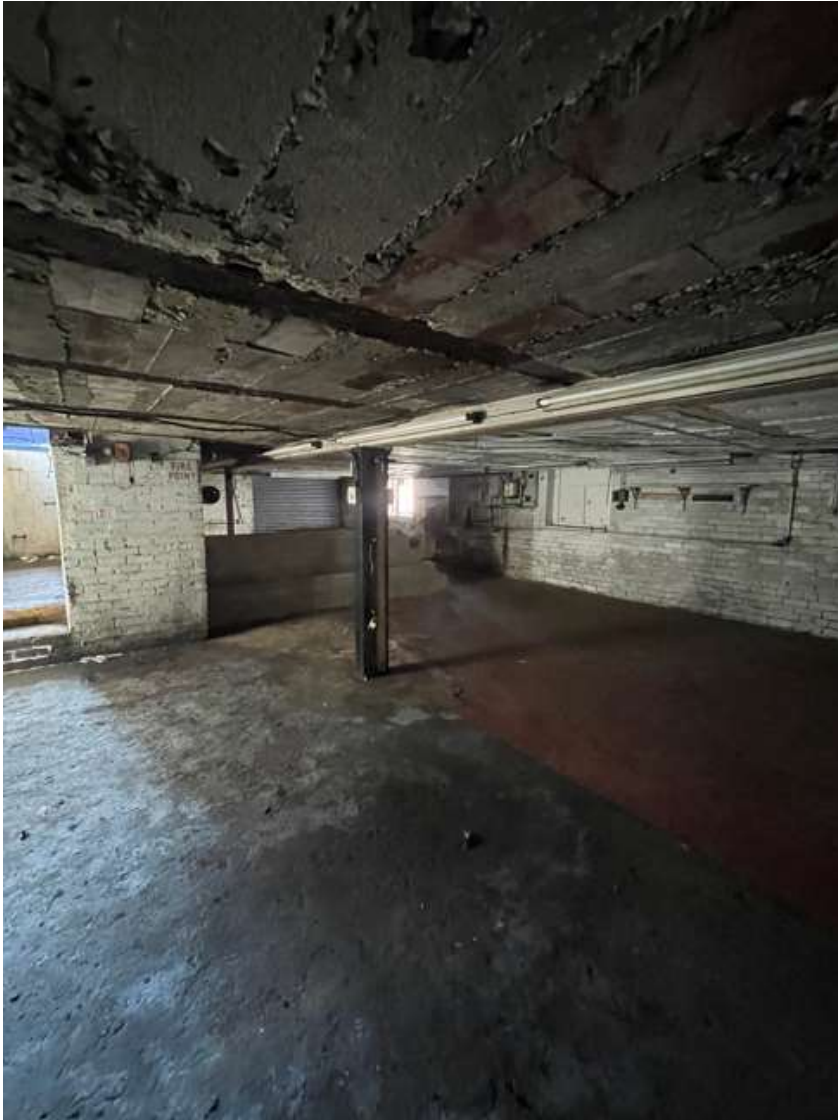
Internal photo of Lower Ground Floor. Floor constructed of steel beams with concrete floor supported between
