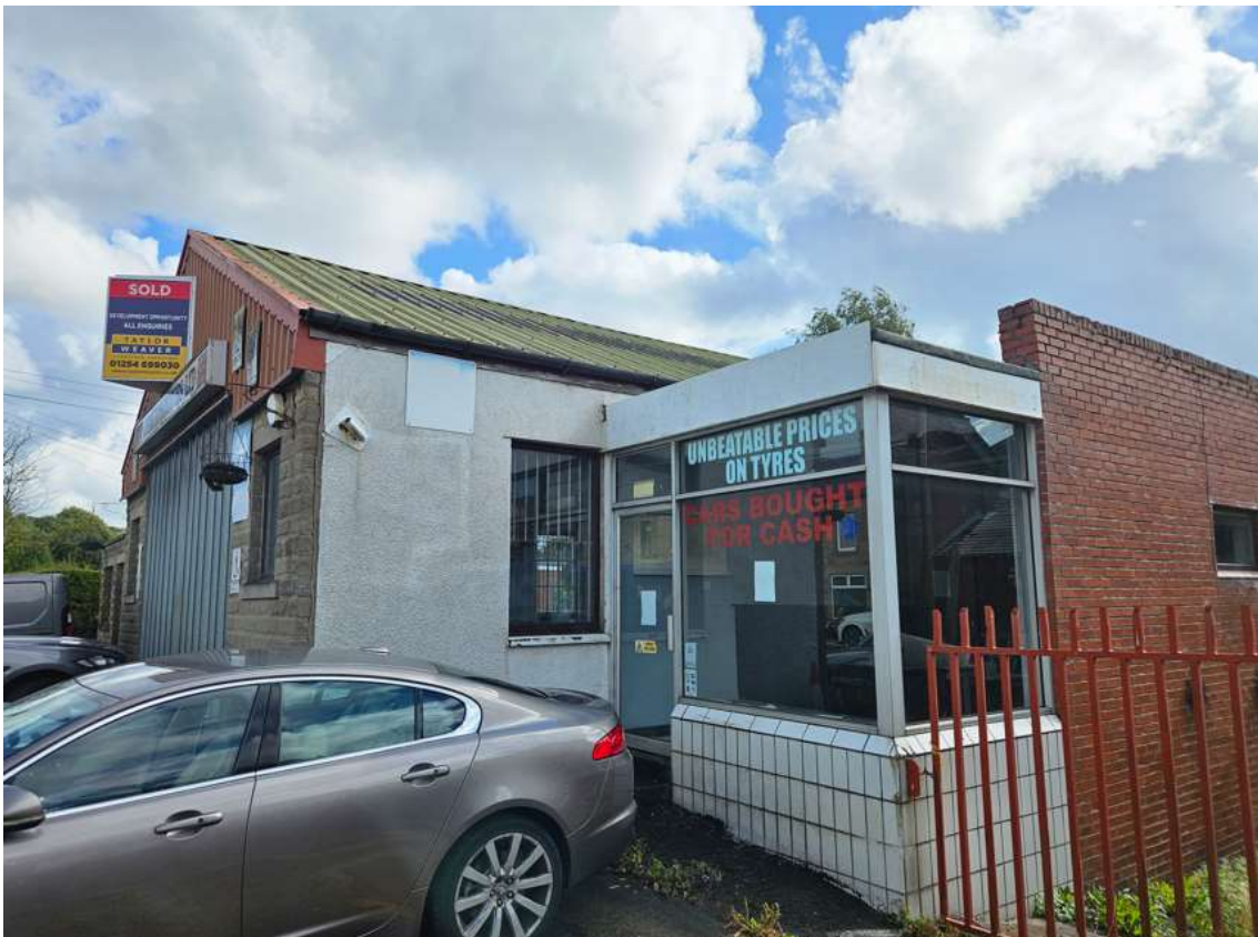
Part front / Side Elevation, showing mix of materials.
