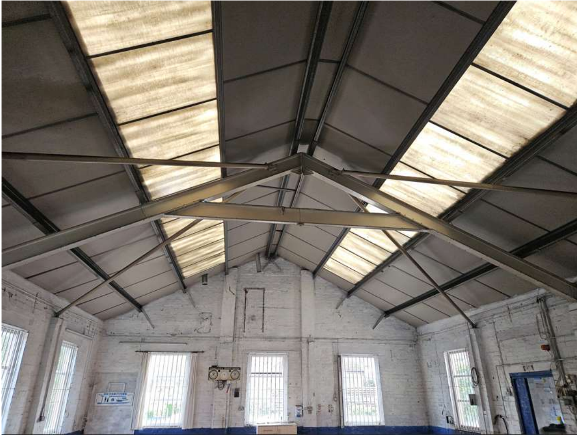
Internal photo of Ground Floor showing steel truss and purlins/ cladding rails supporting profiled roof cladding. Painted brickwork internally.
