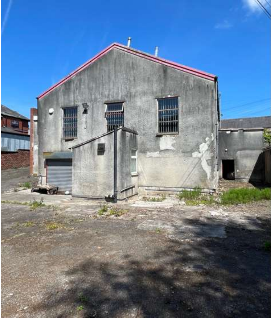
Rear Elevation showing rendered masonry finish.
