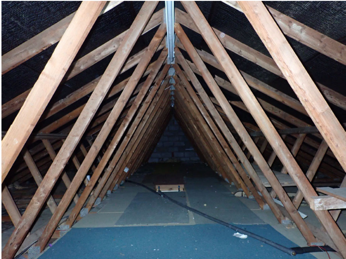
3.2a – The roof void.
