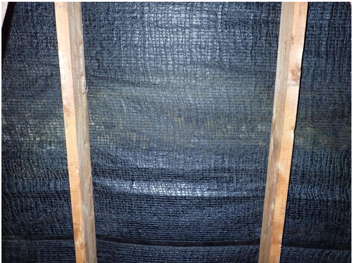
10 – Roof lining is in good condition with no gaps or tears.
