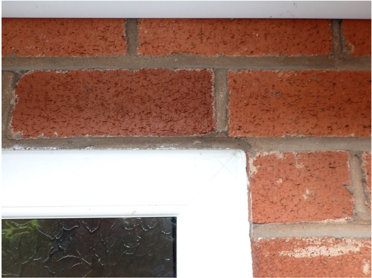
7 – Window and door frames are tightly sealed into brickwork with no suitable gaps.
