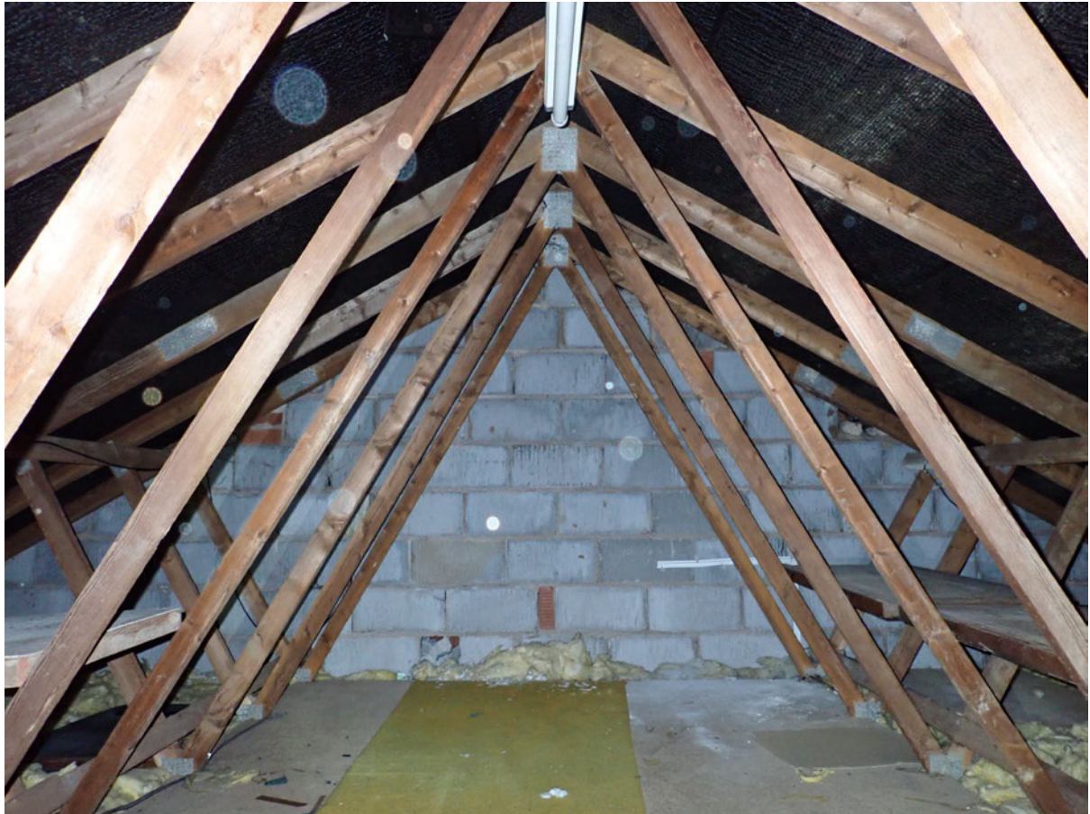
9 – The house has a single roof void.
