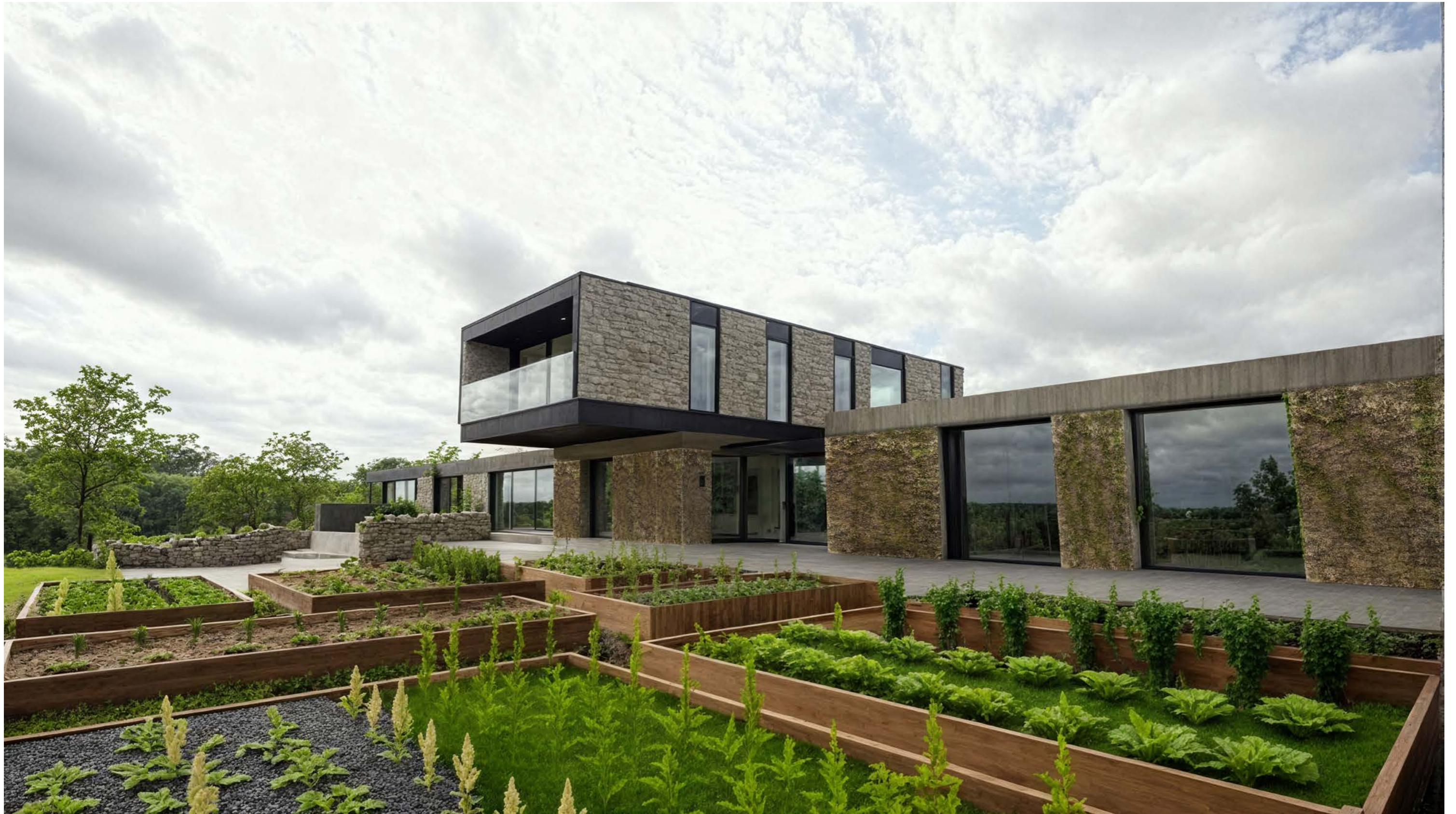
Aerial from within the production kitchen garden showing the cantilevered upper volume.
