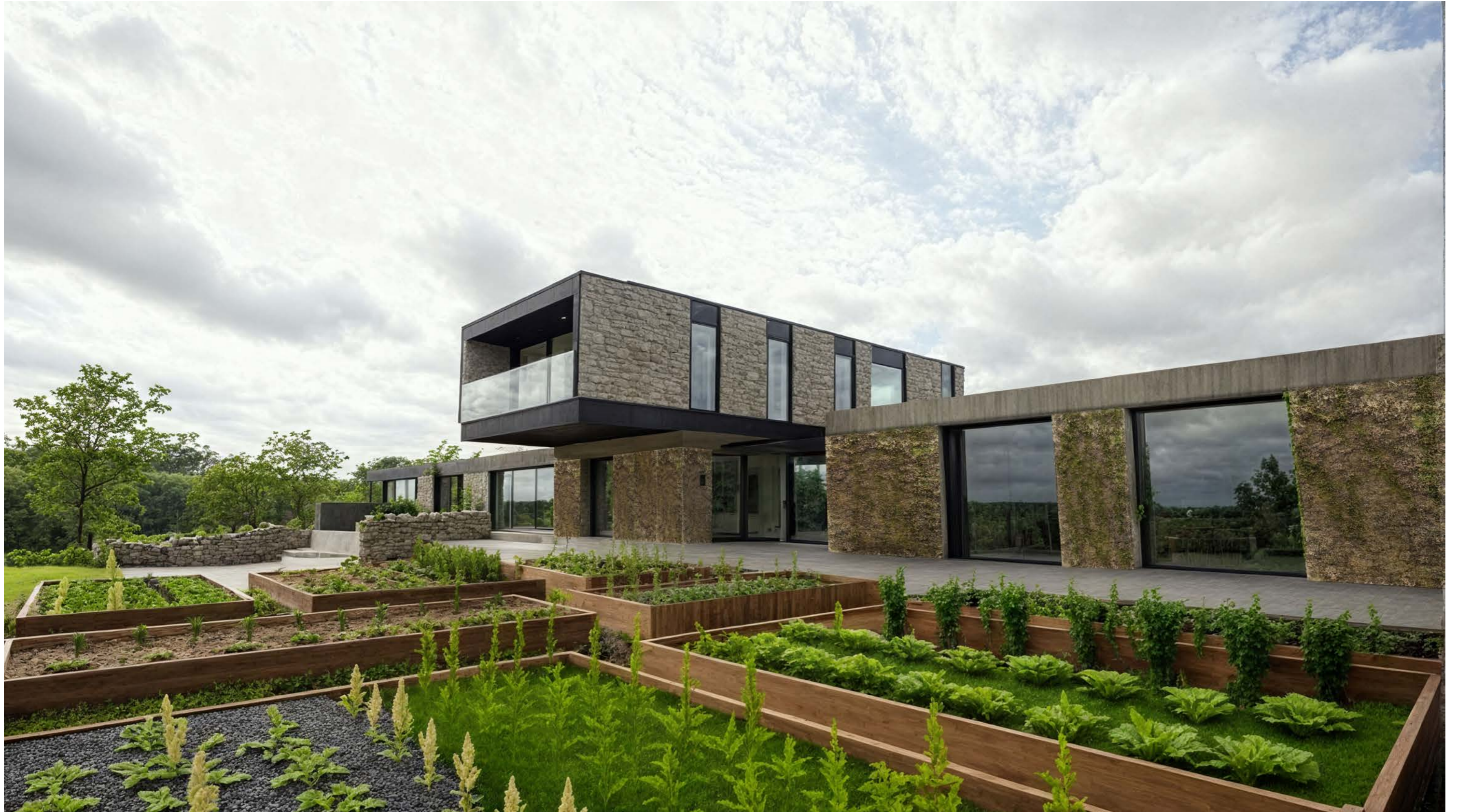
Aerial from within the production kitchen garden showing the cantilevered upper volume.
