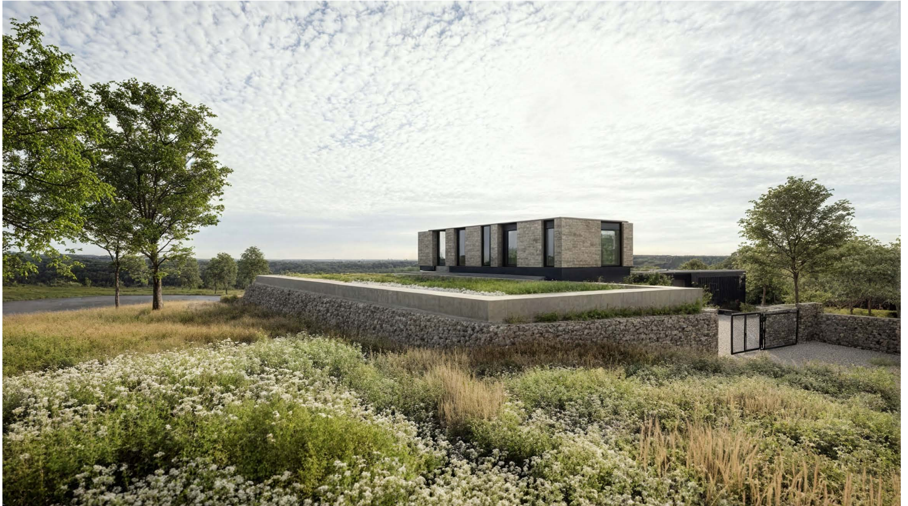
View looking south / west showing upper gabion volume
