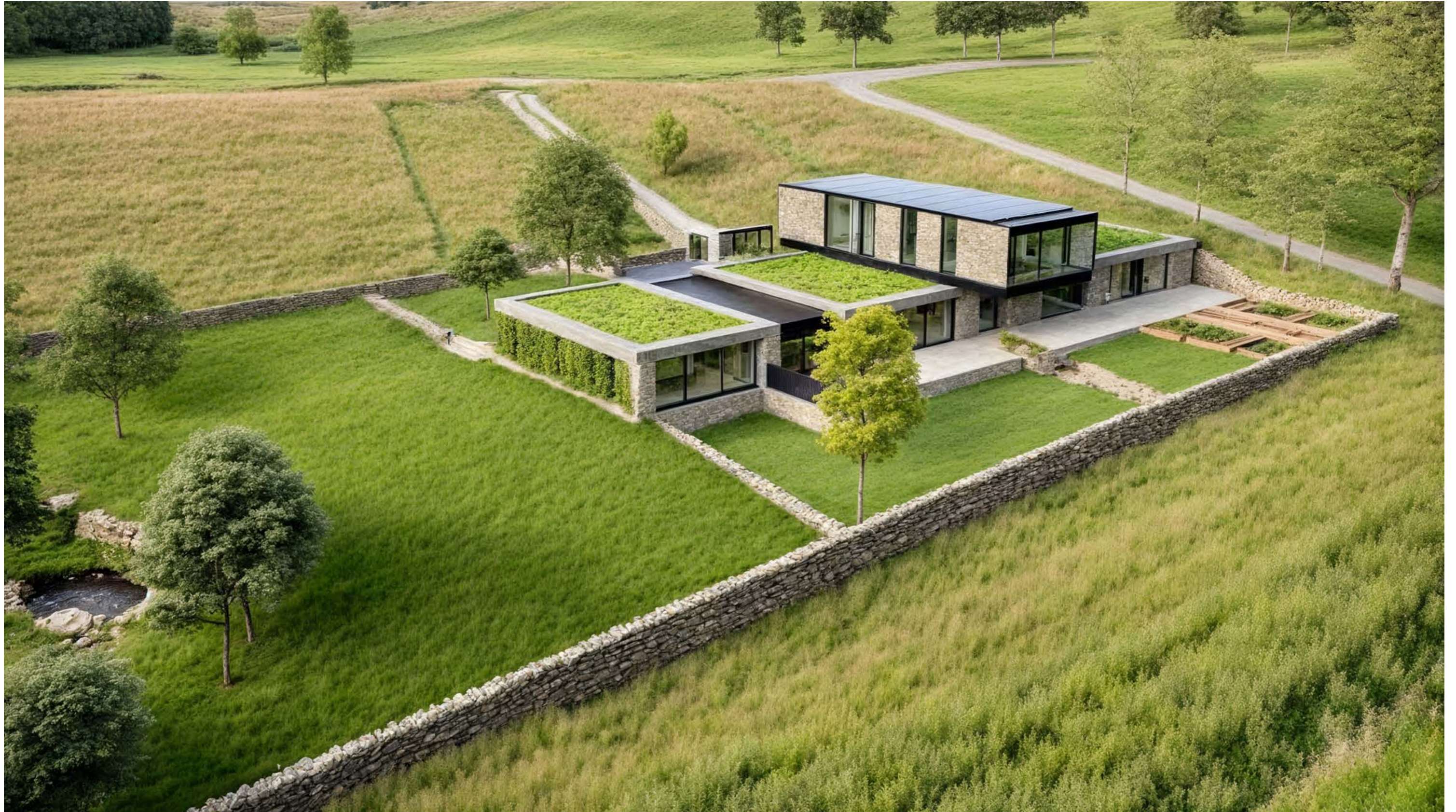
Aerial view looking north east back towards Higher Road.
