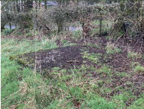
P3: Hardstanding concrete slab located in the north of the site
