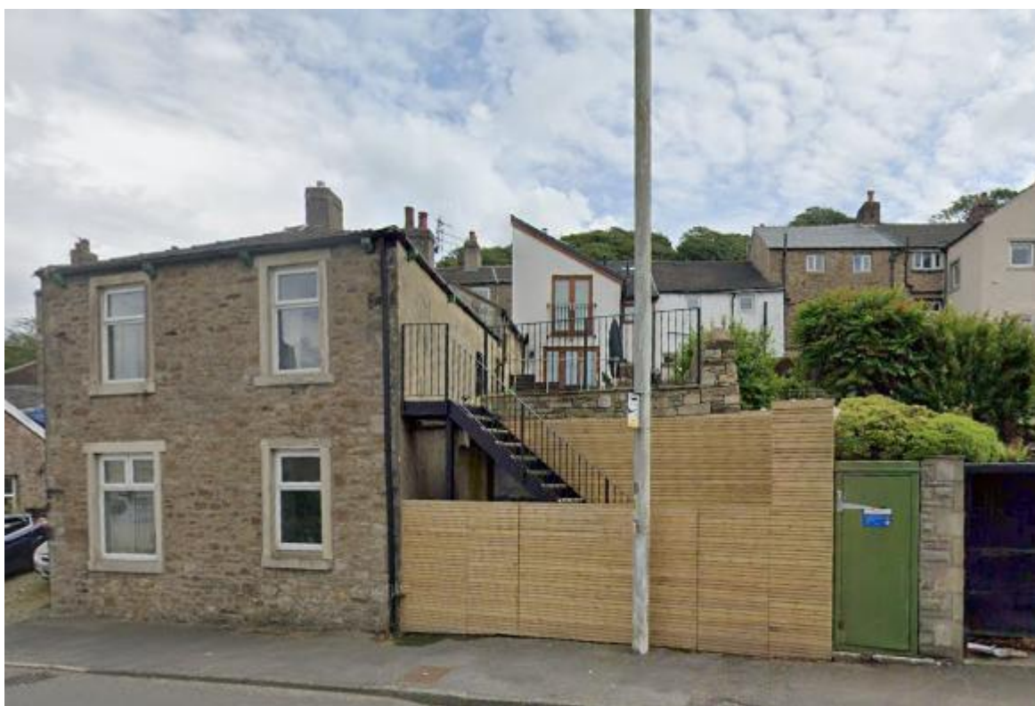
Figure 8. Many nearby properties have raised terraces / balconies and the proposed development would assimilate within such a context
