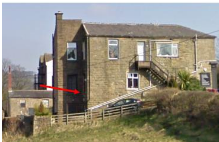
Figure 5. The presence of the proposed balconies does not give rise to undue overlooking concerns as they would be contained within the property's rear outrigger
