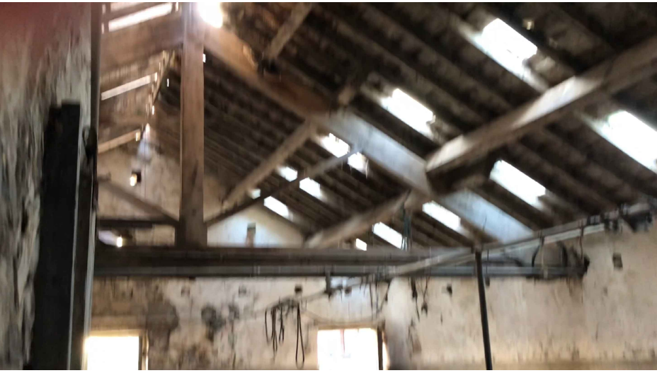
Existing photograph showing original rooflights in lean-to roof prior to re-roof (now blocked up)
