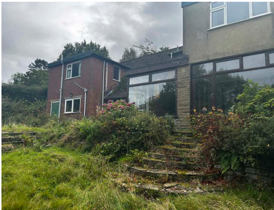
Rear elevation, terracing and steps.
